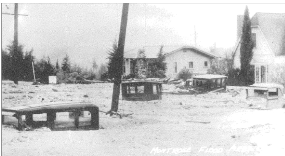
Figure 2.11 Most damage was caused by mudflow (image: HSCV)
