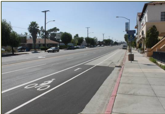
Maintaining the existing Class 2 dedicated bicycle lane along Foothill Boulevard is supported, as it is an important link in the region's bicycle network.
