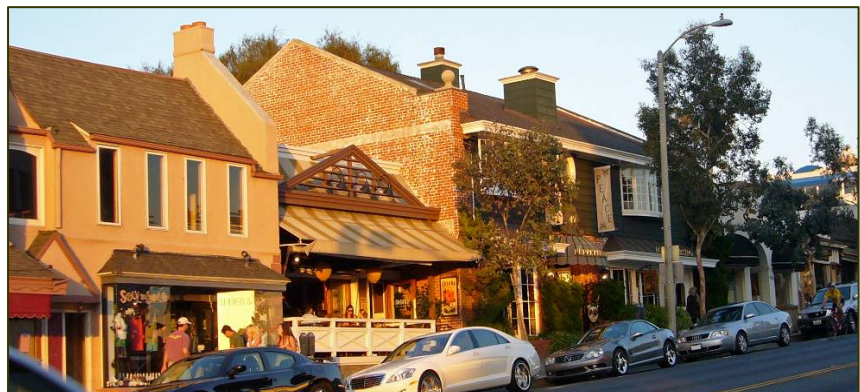
Buildings at the property line with active street frontages provide pedestrian orientation
