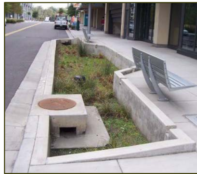
Parkway landscaping with drainage swales are supported along the Verdugo Boulevard right-of-way.
