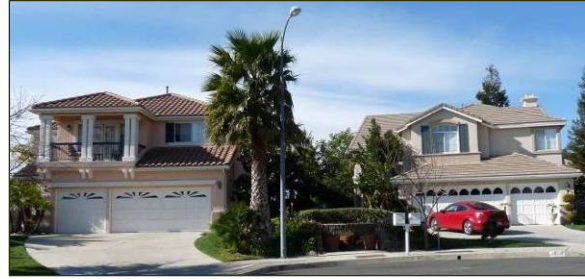
Houses in Markridge have similar one- or two- story porticos and front-facing 3-car garages
