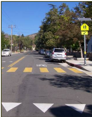
Safe Routes to School enhancements including zebra striped crosswalks and sharrows help promote bicycling and walking.
