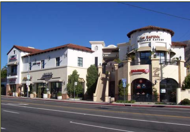
The building at Foothill and Pennsylvania features a variety of roof heights and forms, from gabled ends, hipped roofs, flat parapets and a circular rotunda.
