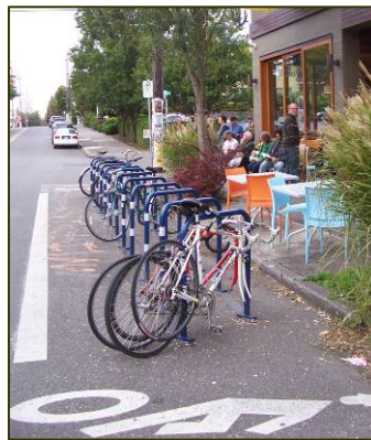
The installation of bike corrals should be considered to further enhance accessibility for those traveling by bicycle.
