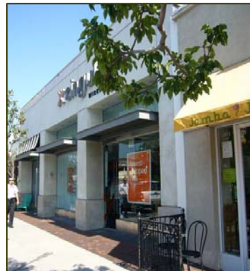
Recessed storefronts and canopy design provide quality detailing
