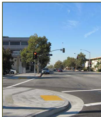
Curb extensions at crosswalks are supported along Foothill Boulevard to increase safety and enhance mobility for all users.
