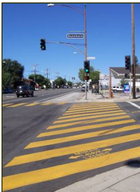
Enhanced crosswalks at intersections along Foothill Boulevard increase visibility and safety for pedestrians.
