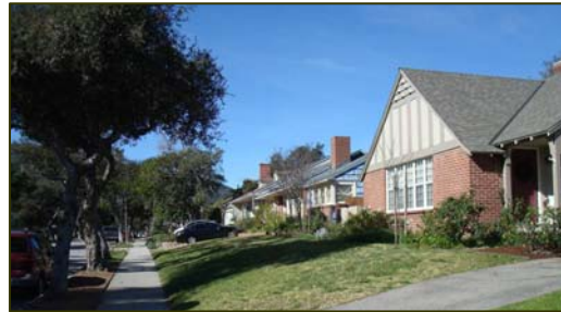
Dwellings should present a simple and pleasing composition using a common vocabulary of forms.
