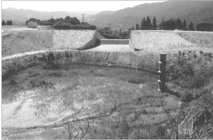
Figure 2.13 Upstream view of typical debris basin (image: HSCV)
