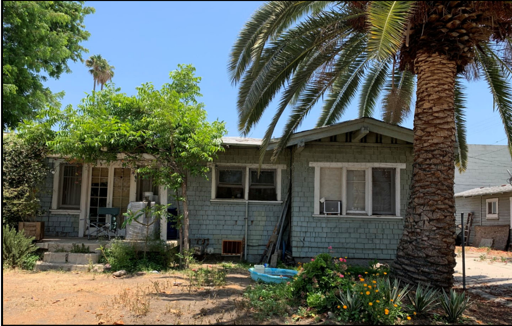
Figure 3.1.2. Southeast end of southwest façade of 1642 South Central Avenue, view facing northeast (SWCA, June 2021).
