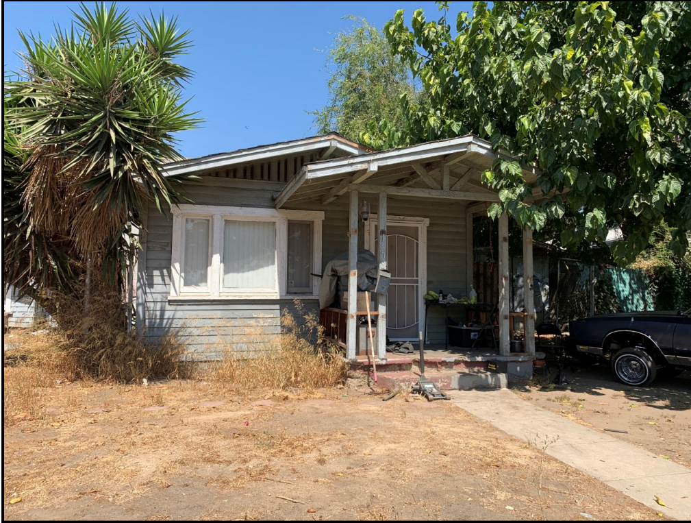
Figure 3.1.4. Southwest (primary) façade of 1608 Gardena, view facing northeast (SWCA, August 2021).
