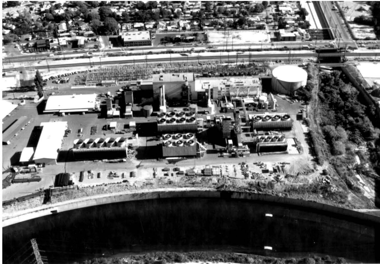
GRAYSON POWER PLANT
