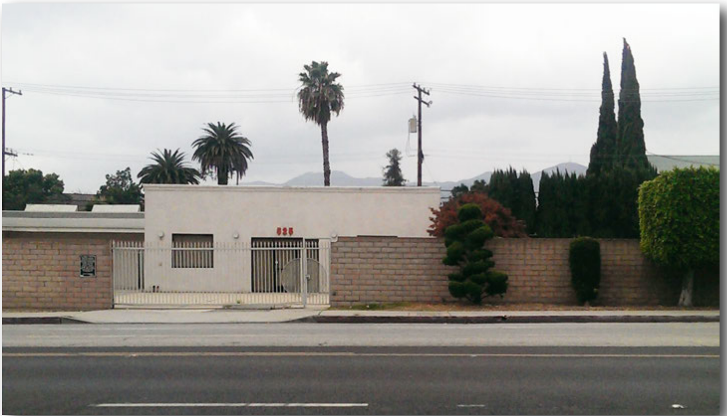
Located along the southern frontage of W. Colorado St. looking north towards the Project site
