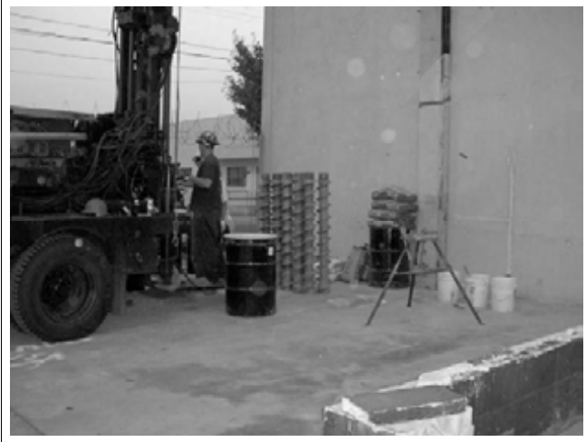
8. View of the installation of MW-1.
