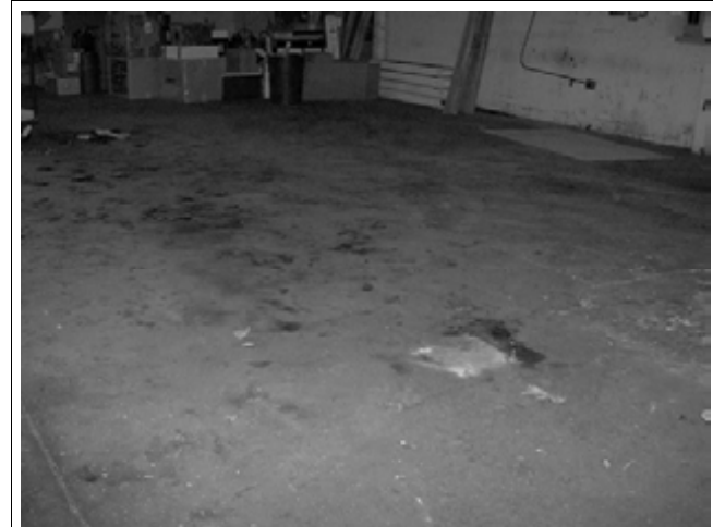
1. View of typical ink staining on the floor of Building 4, the former Glendale Rotary Offset Printing.
