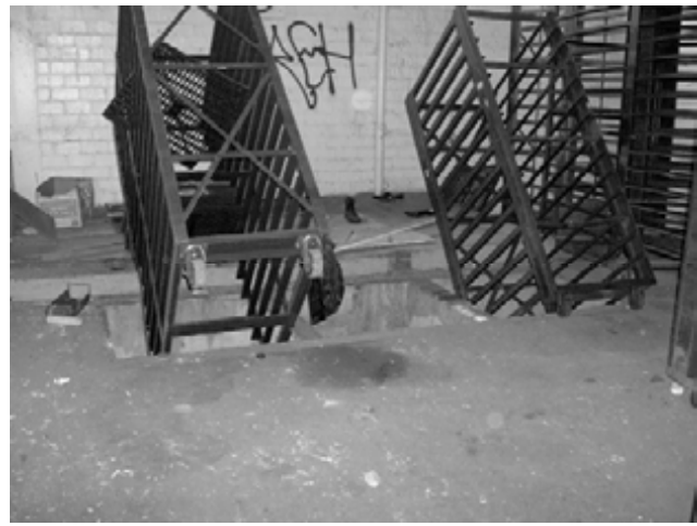
4. View of the three-stage clarifier in Building 1.
