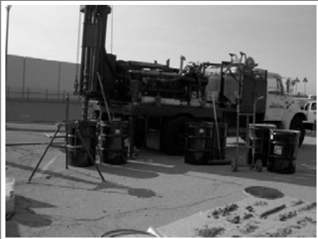
7. View of the installation of MW-3.
