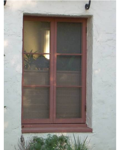
External grids add texture and detail to windows
