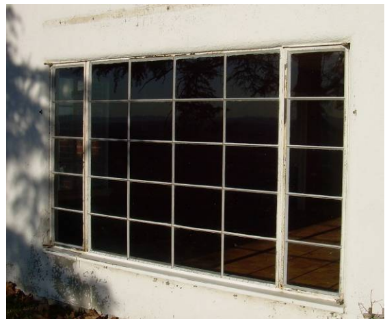
Stucco bullnose at top and sides of opening
