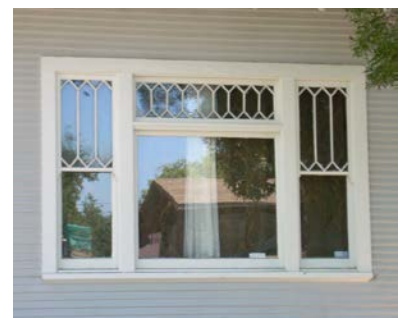
Internal grid does not recall appearance of true divided-light window
