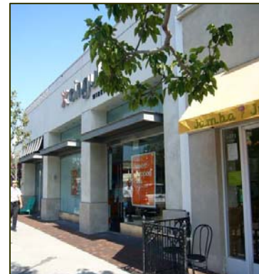
Recessed storefronts, storefront and canopy design provide quality detailing
