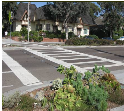
Pedestrian amenities at crosswalks such as curb extensions and median refuges will enhance safety for all users.
