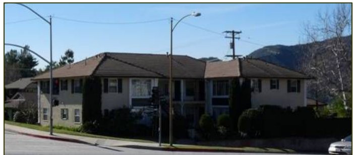
The series of Ranch-style apartment buildings arrayed along Valihi Way and Stancrest Drive represents an unusually cohesive grouping of multi-family structures in the Ranch style. In scale, they are often reminiscent of single-family houses, but typically consist of duplexes and triplexes, with a few larger buildings containing up to twelve units.
