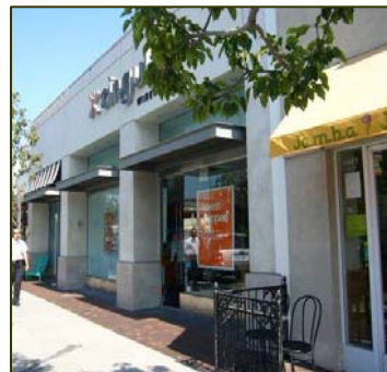
Recessed storefronts, storefront and canopy design provide quality detailing
