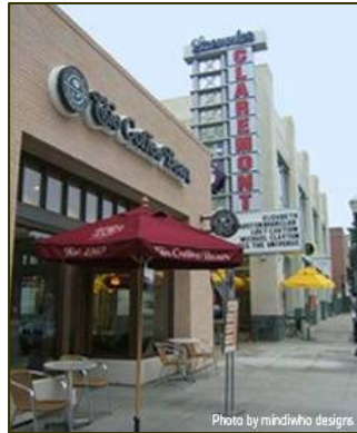
Create active street front environment that provides color texture and variation in building plane
