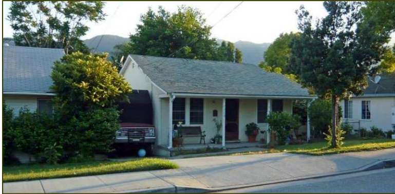
There is variety in buildings and streetscape throughout Verdugo City
