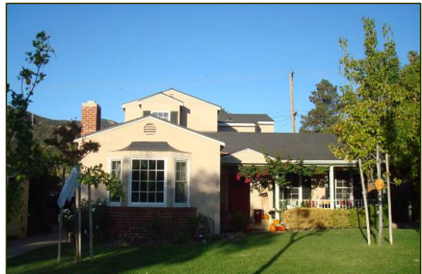
Consider setting back a new second story from the front face of the ground floor, to prevent a massive appearance.
