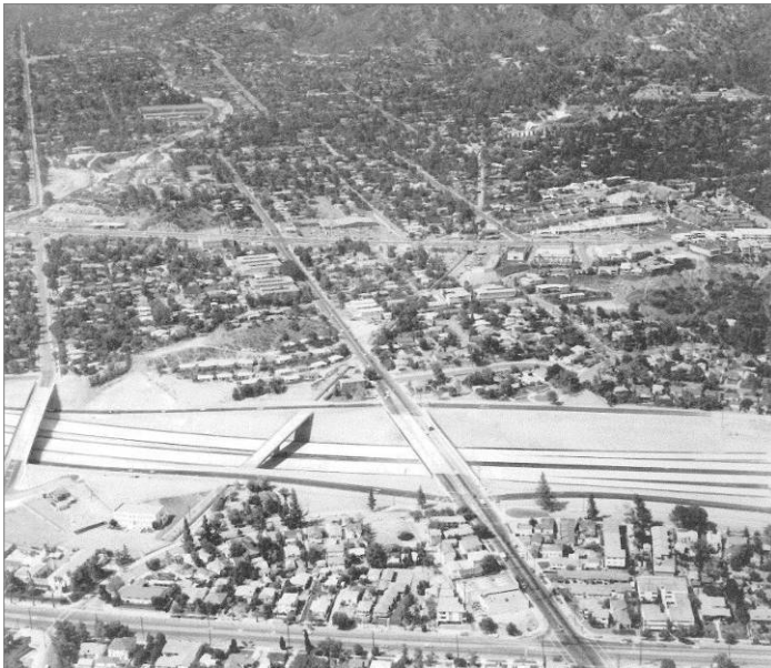
Figure 2.14 210 Freeway in 1972, just prior to opening; impact on neighborhood is evident (image: GPL)
