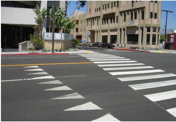
Figure 5-11. Zebra stripe crosswalk with yield line on Colorado St.
