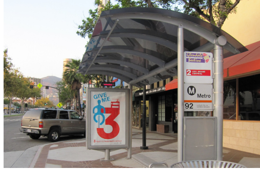
Figure 5-16. Bench and shade structure at Brand Blvd. bus stop
