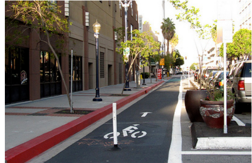
Figure 5-22. Protected bike lane, Long Beach, CA
