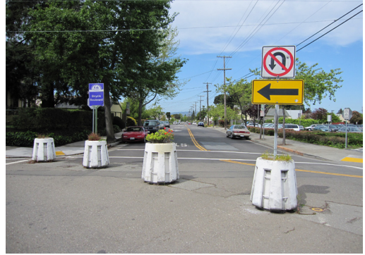
Figure 5-2. Diverter in Berkeley, CA
