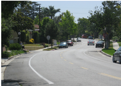
Figure 5-3. Painted edge line
