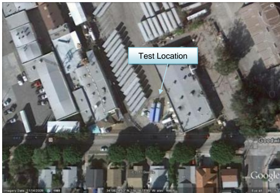
FIGURE 7 - WBA TEST LOCATION AT GS-3
