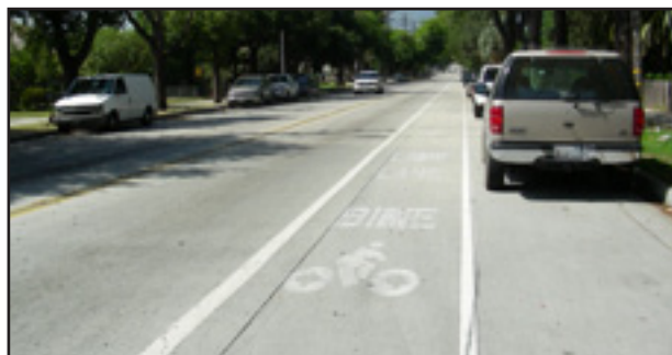
Figure 8-3: Bike Lane Striping and Stencil
