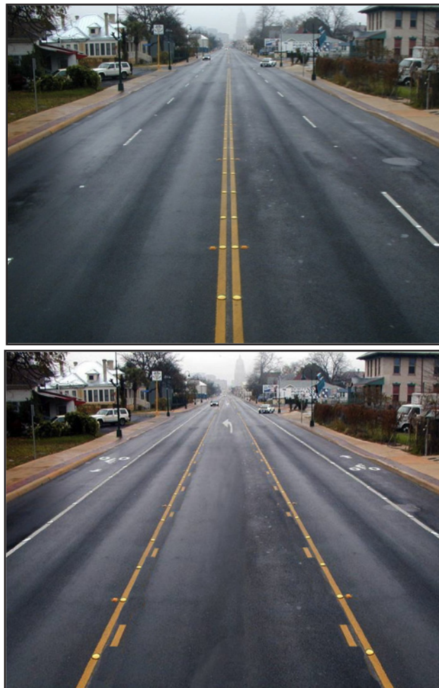
Figure 8-28: Before and After Road Diet
