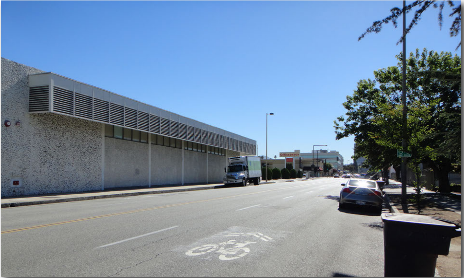
Located on south side of Broadway looking east past the Project site
