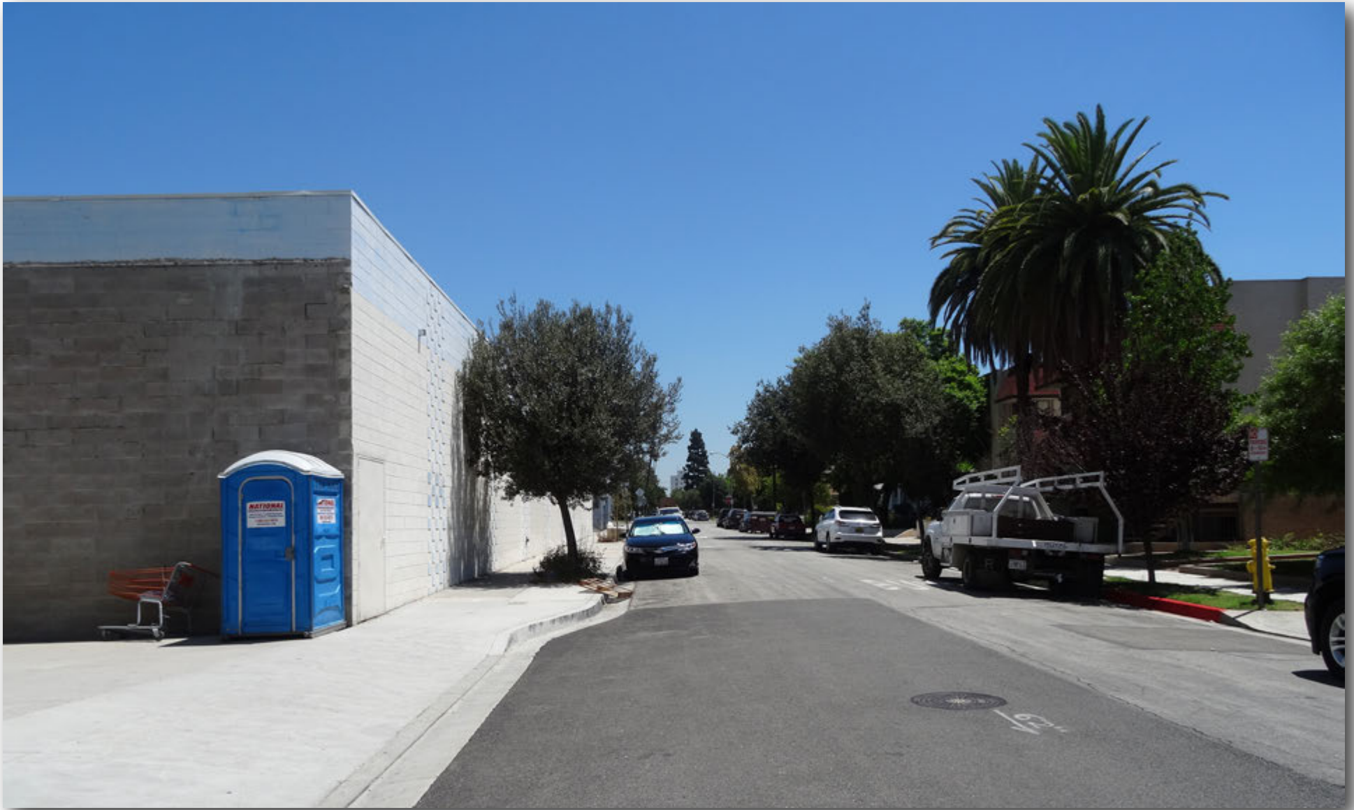
Outside Project site on W. Elk looking east
