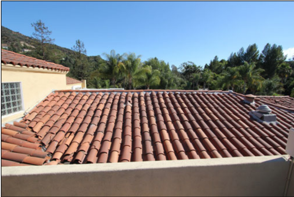
Fig. 42: 3067 E. Chevy Chase Drive, roof, view south (Chattel, 2014)
