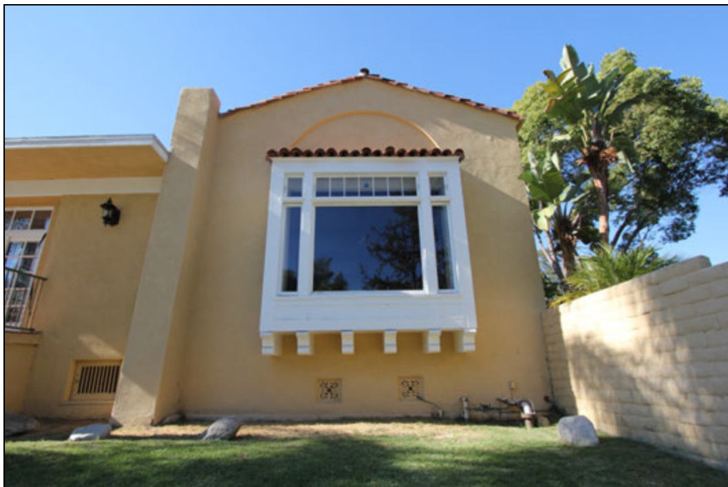
Fig. 39: 3067 E. Chevy Chase Drive, south elevation, view north (Chattel, 2014)
