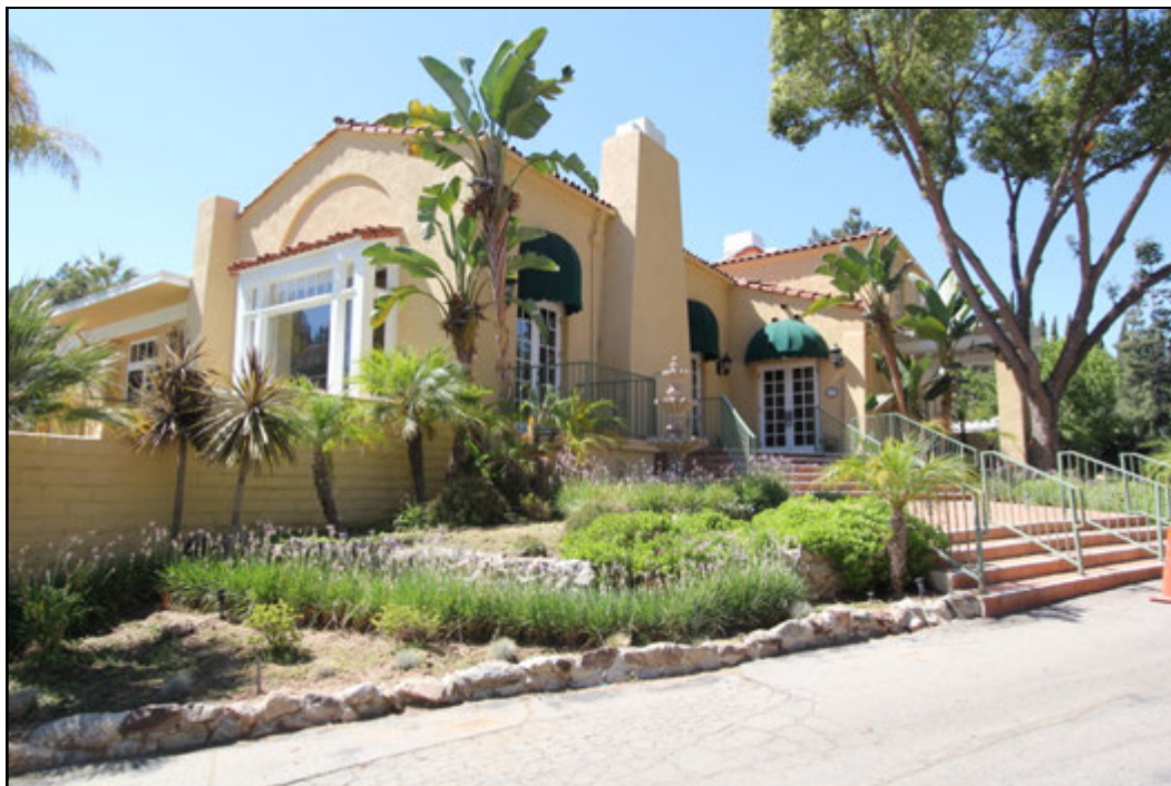
Fig. 19: 3067 E. Chevy Chase Drive, south and east elevations, stairs to east elevation secondary entrance at right, view northwest (Chattel, 2014)
