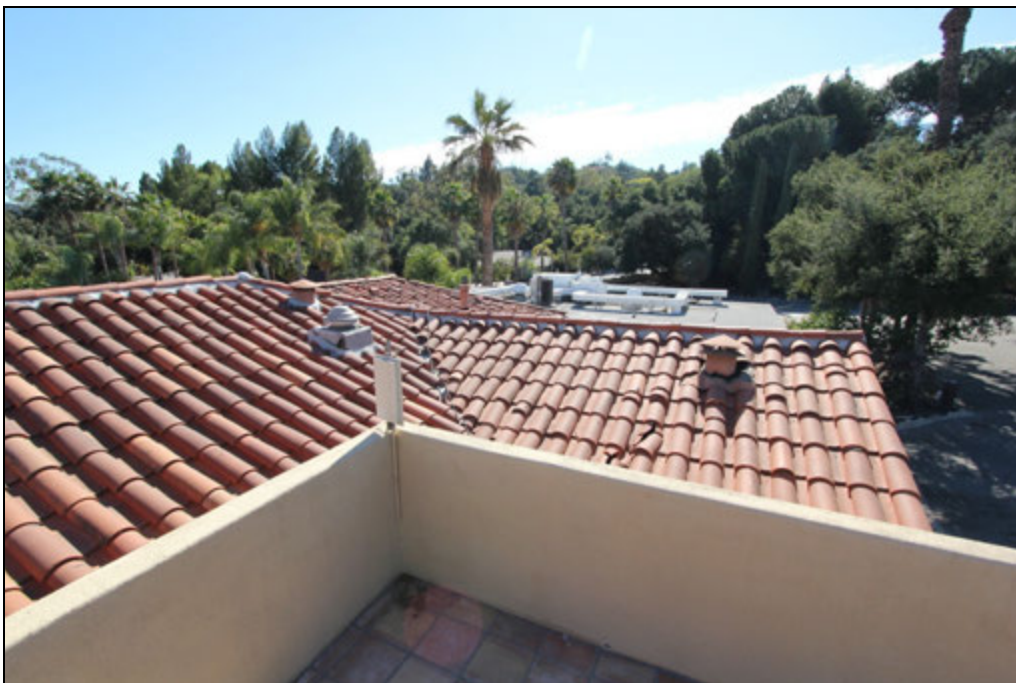
Fig. 43: 3067 E. Chevy Chase Drive, roof, view west (Chattel, 2014)
