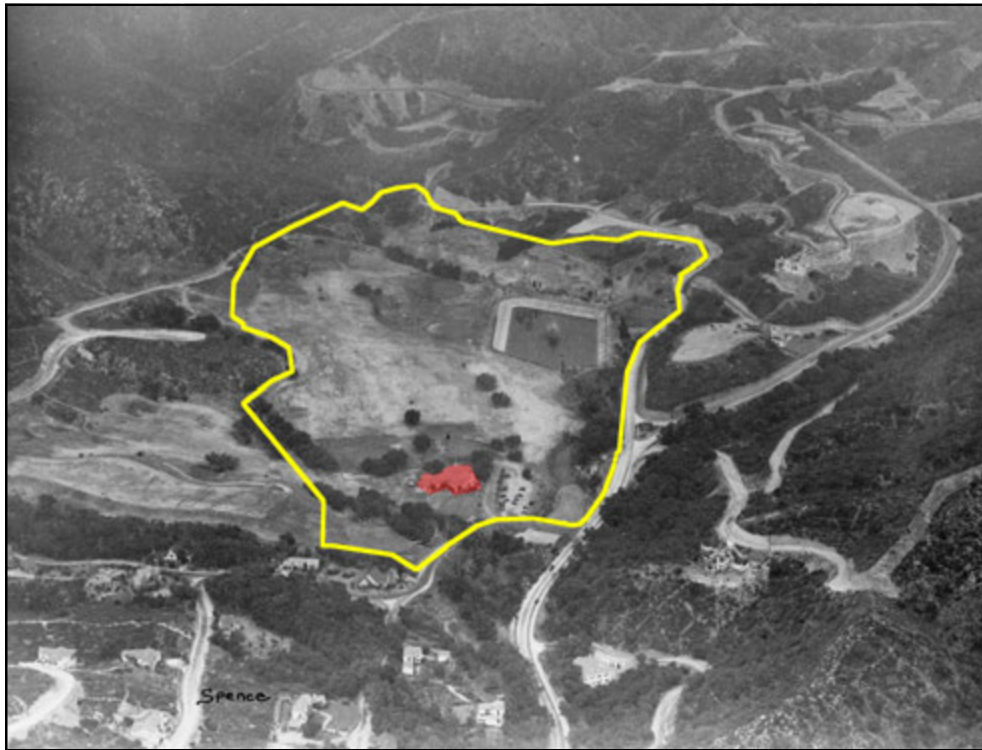
Fig 1: 3067 E. Chevy Chase Drive, historic aerial, Club property outlined in yellow and clubhouse highlighted in red (UCLA, Benjamin and Gladys Thomas Air Photo Archives, Spence, 1930)
