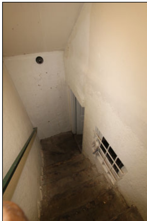
Fig. 71: 3067 E. Chevy Chase Drive, stairs to basement, view east (Chattel, 2014)
