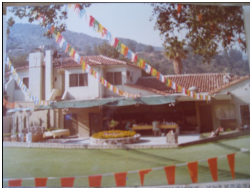
Fig. 13: 3067 E. Chevy Chase Drive, subject property north elevation, view south (Chevy Chase Country Club, 1975)
