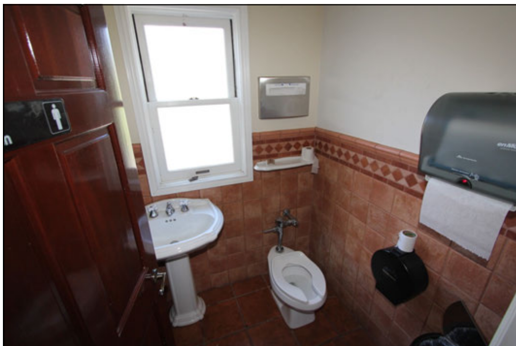
Fig. 77: 3067 E. Chevy Chase Drive, second floor, men's restroom, typical, view north (Chattel, 2014)
