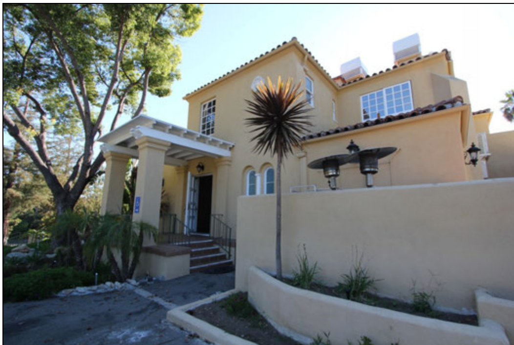
Fig. 23: 3067 E. Chevy Chase Drive, east and north elevations, view southwest (Chattel, 2014)
