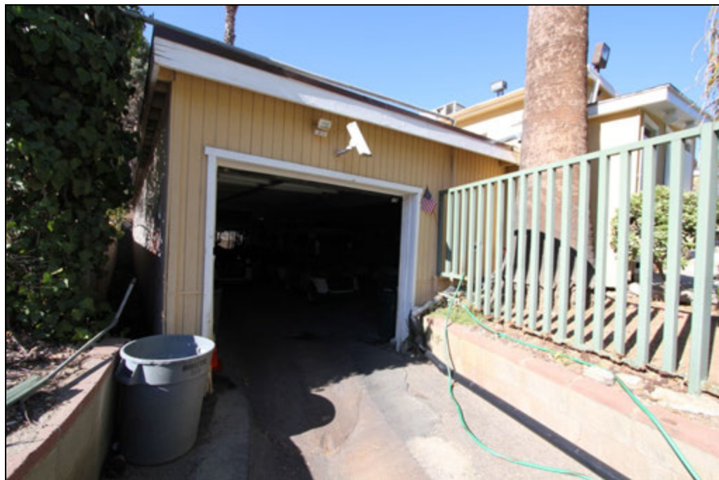
Fig. 33: 3067 E. Chevy Chase Drive, garage south entrance, view north (Chattel, 2014)
