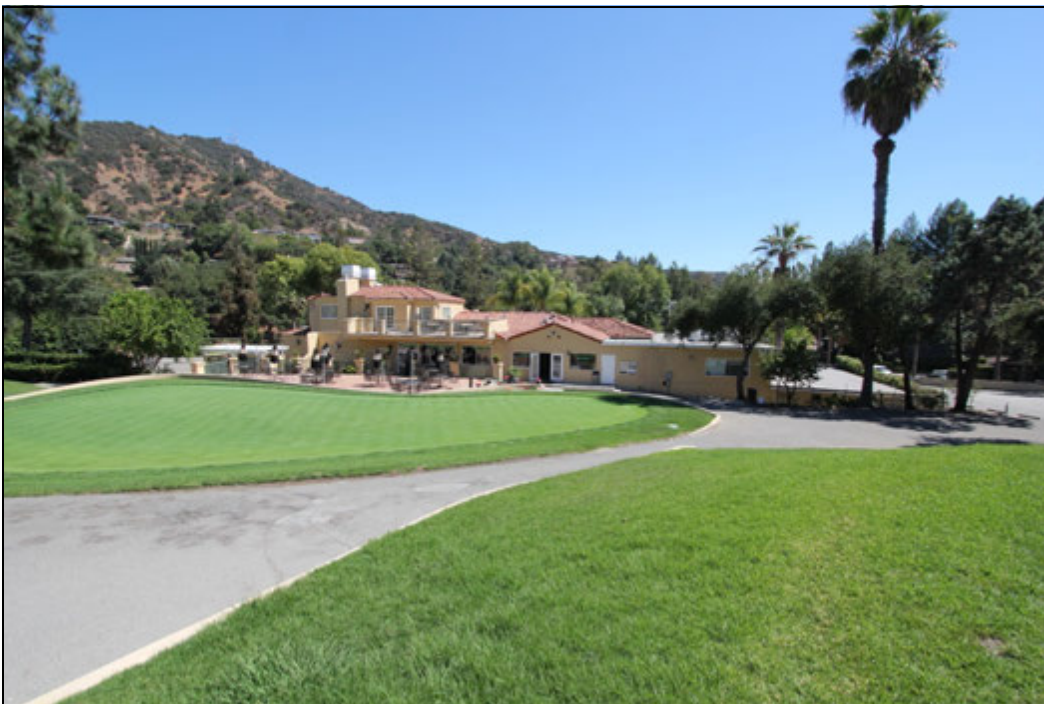
Fig. 29: 3067 E. Chevy Chase Drive, north elevation, golf course in foreground, subject property in background, view south (Chattel, 2014)
