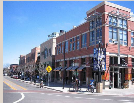
ABOVE: Boulder's public shared parking garage wrapped in retail and office space.
