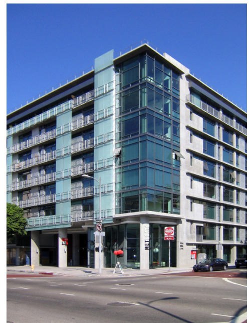
BELOW: The Met Lofts in Downtown LA.
