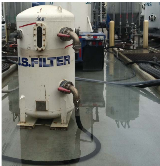
Figure A.1 Resin preconditioning vessel
