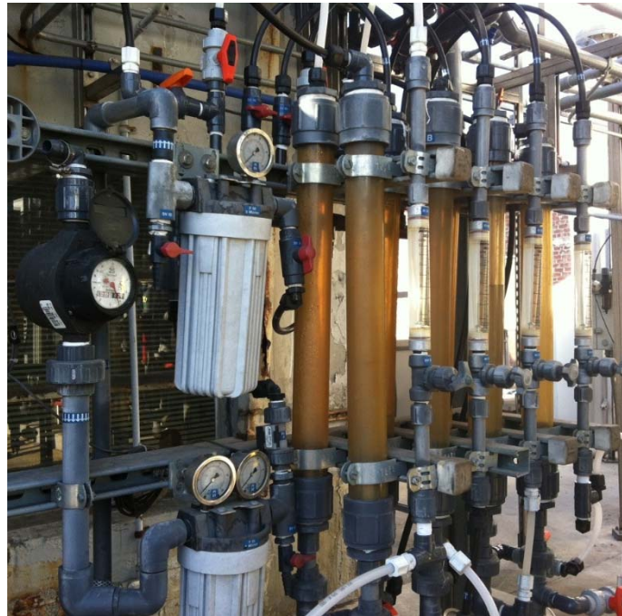
Figure A.2 Photograph of small columns used for resin holding test
