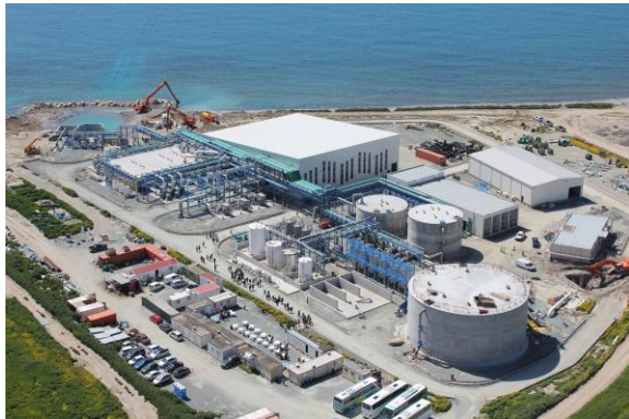
Figure 2.18: Seawater Desalination Plant
