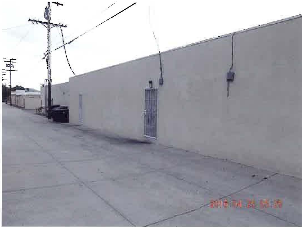
BLDG REAR SIDE, NORTH WALL. From alley.
