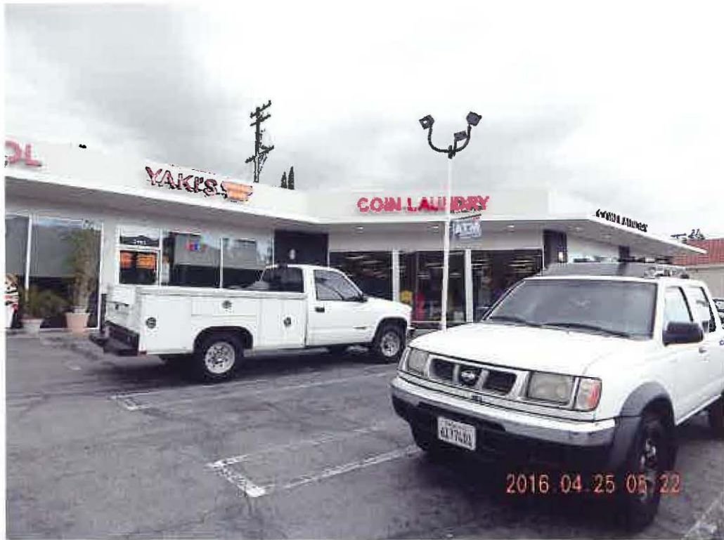
BLDG. SOUTH SIDE, from parking looking at north-east
