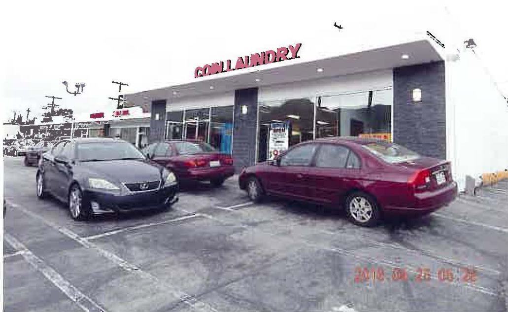
BLDG. SOUTH-EAST CORNER, from side parking.
