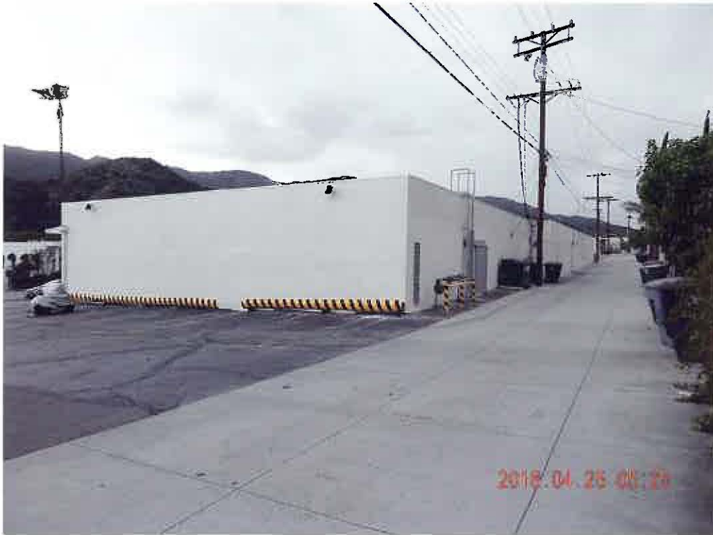
EAST WALL VIEW, from alley.
