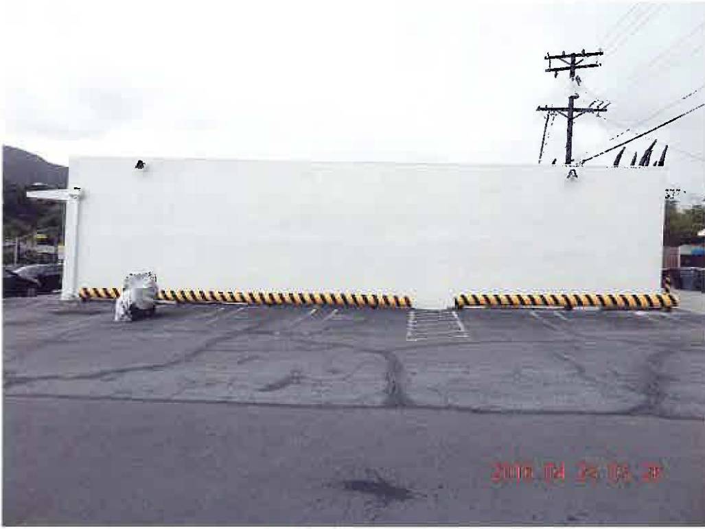
EASR WALL VIEW, from parking.
