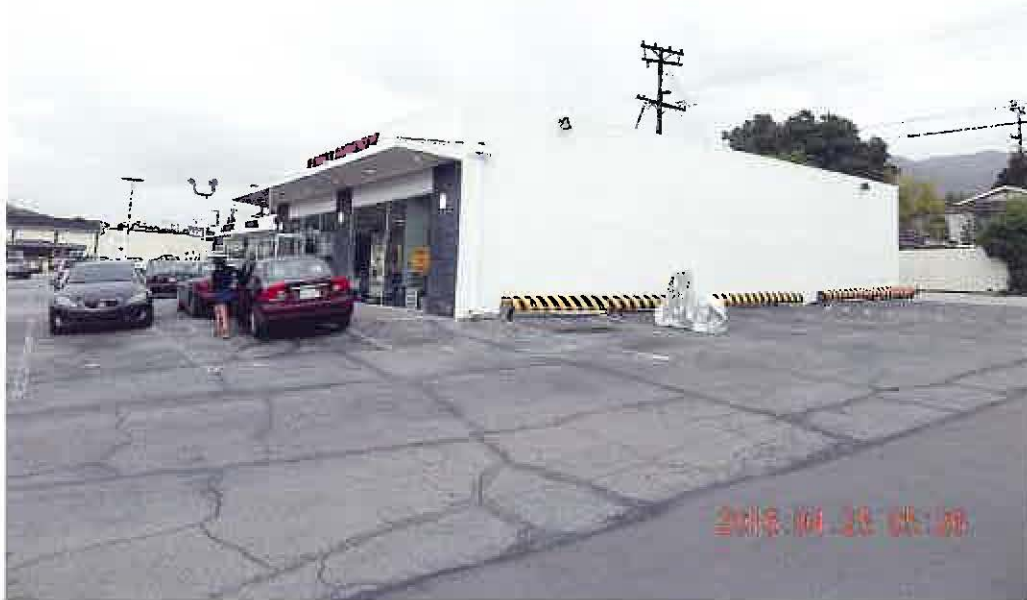
BLDG. SOUTH-EAST CORNER, from side parking.
