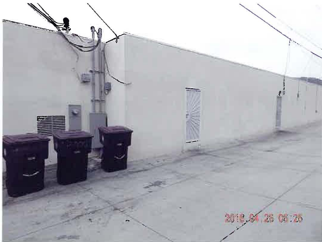
BLDG REAR SIDE, NORTH WALL. From alley.
