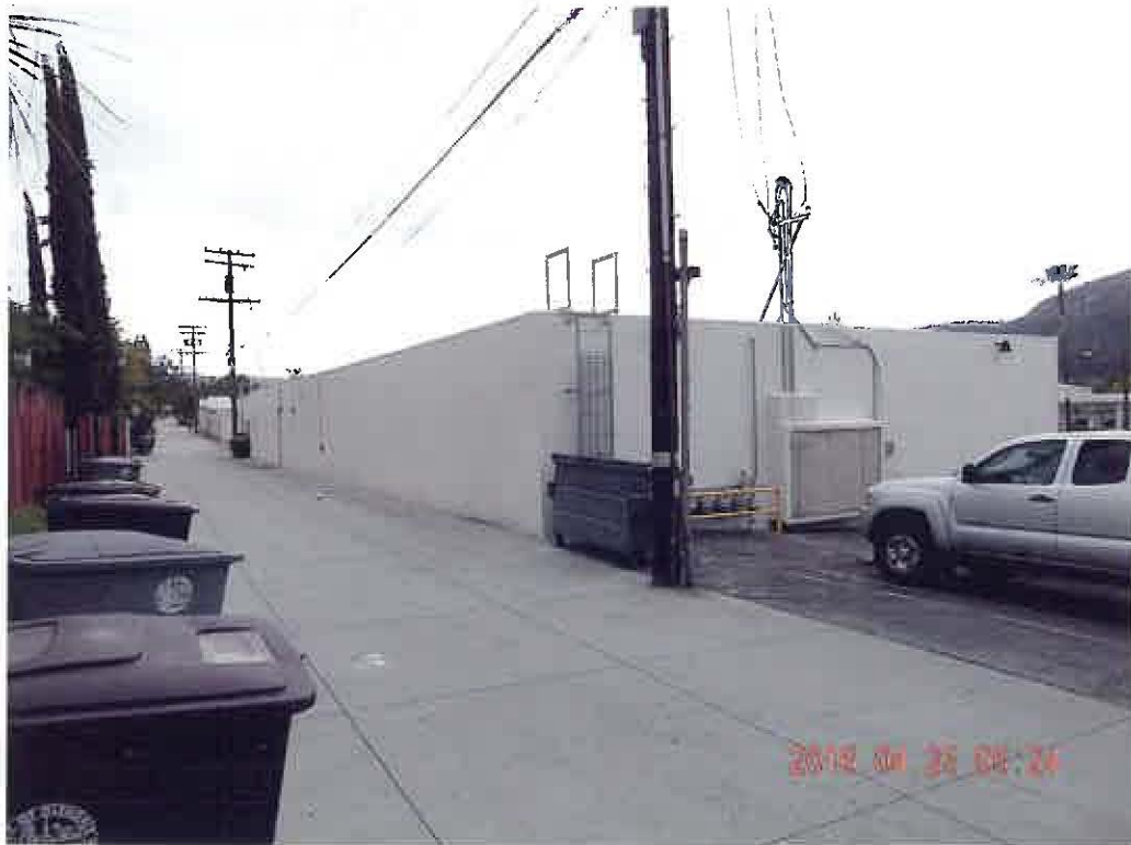
BLDG. NORTH-WEST CORNER, from the alley.
