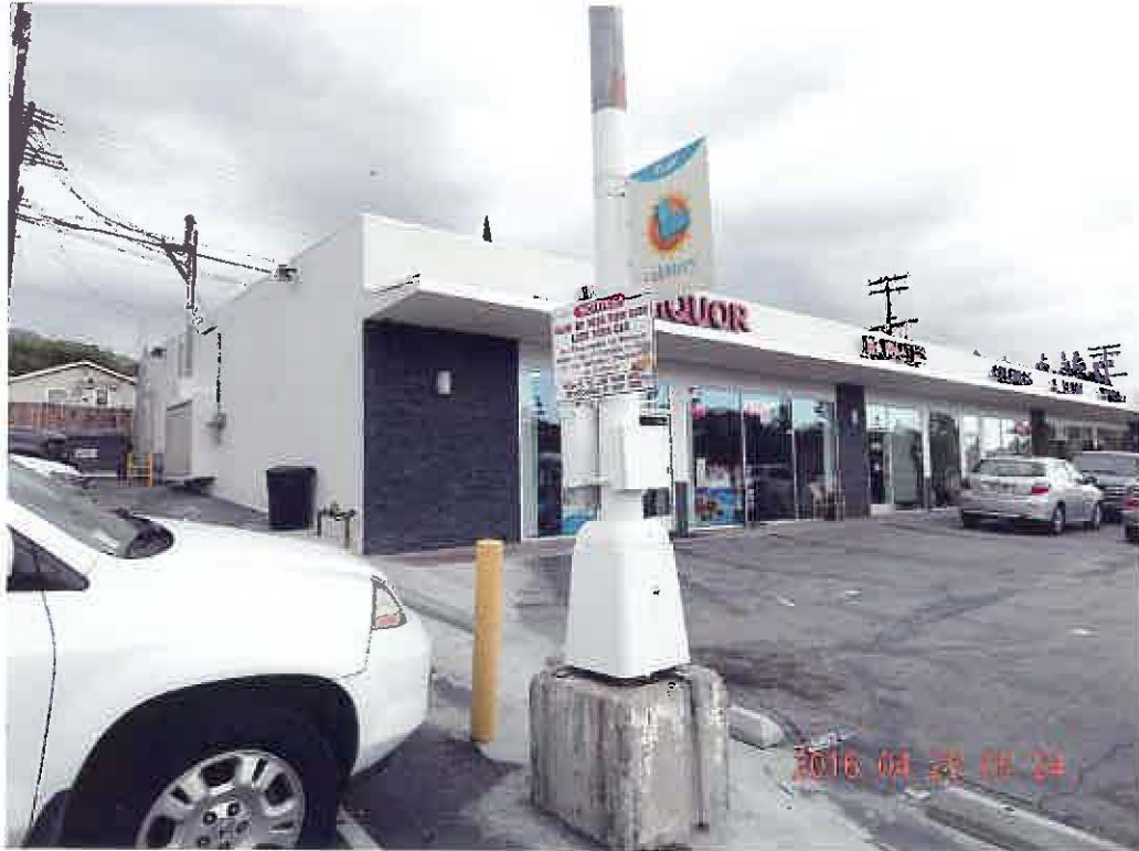
BLDG. SOUTH-WEST CORNER.
