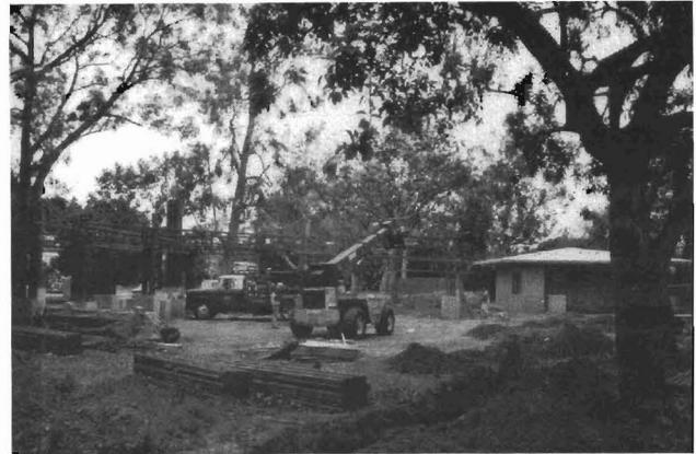
Palmer Park Renovation
