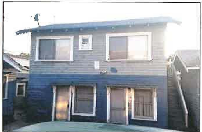
Two-story residence (350A, 350B, and 350½ Salem Street), façade, view to the west (2017)
