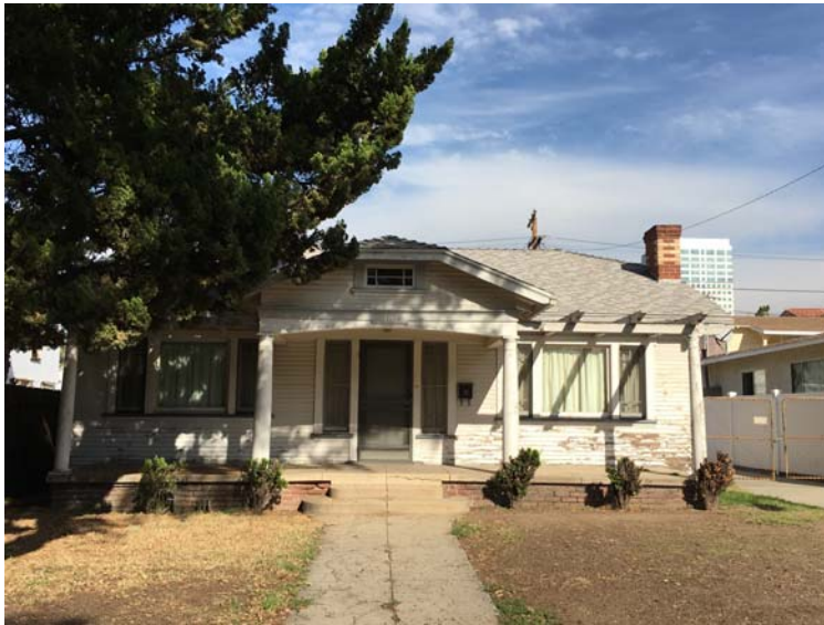
Figure 1. View of the Primary Façade, Facing North SOURCE: Sapphos Environmental, Inc., 2016
