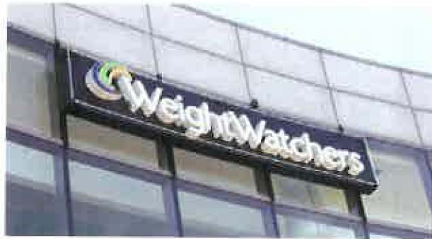
EXISTING WEIGHT WATCHERS WALL SIGN TO BE REPLACED (EXISTING SIGN: 14'-6"W x 7"D x 2'-8"H)
