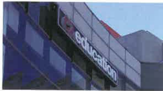
EXISTING C2 EDUCATION WALL SIGN TO BE REPLACED (EXISTING SIGN: 15'-6"W x 8"D x 2'-8"H)
