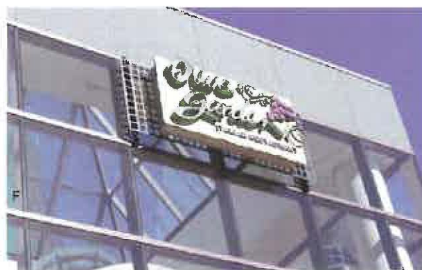
EXISTING OLIVE GARDEN WALL SIGN TO BE REMOVED AND RELOCATED (EXISTING SIGN FRAME & BOX: 10'-6"W x 9' D x 4'-3"H)
