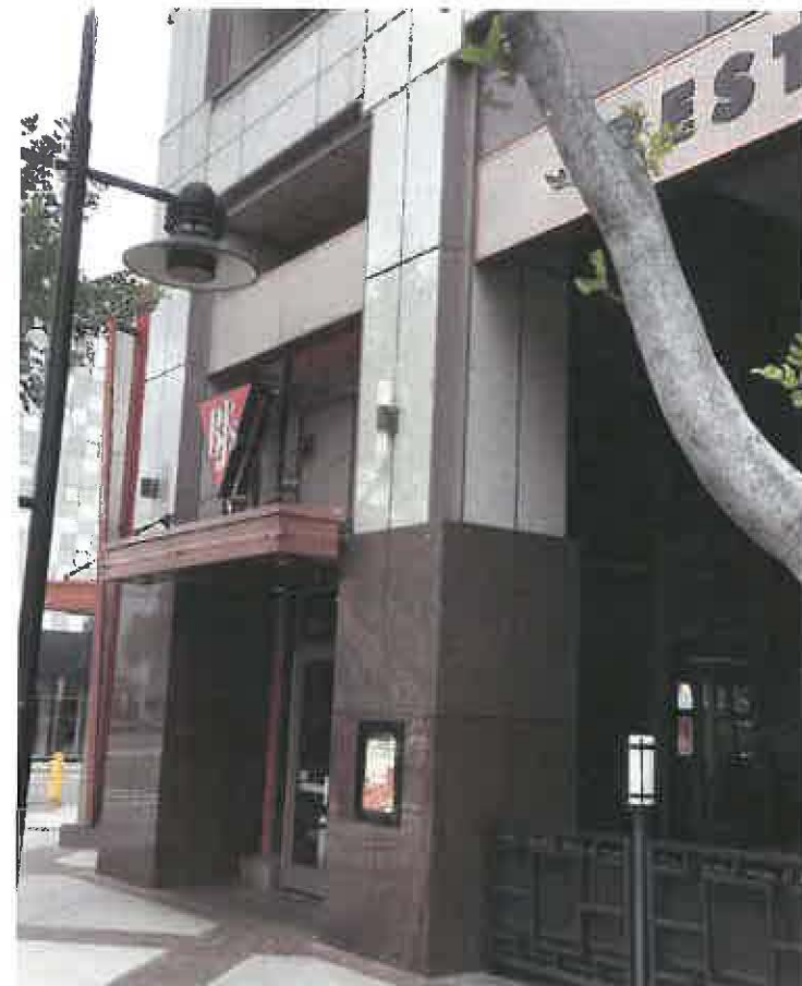
Existing signs on N Brand Boulevard
