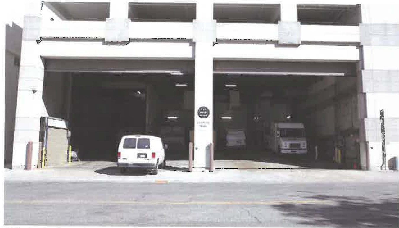
Existing loading Dock entrance sign on Orange Street
