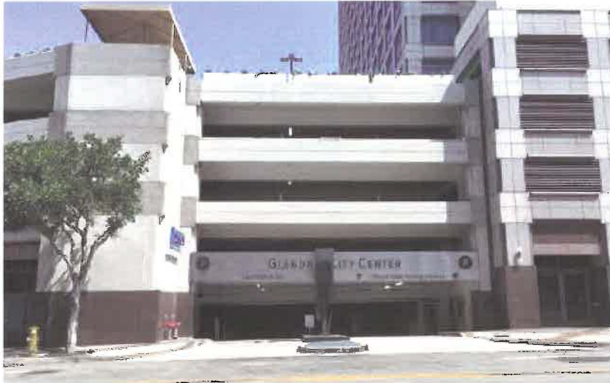
Existing parking garage entrance ID sign on W Broadway
