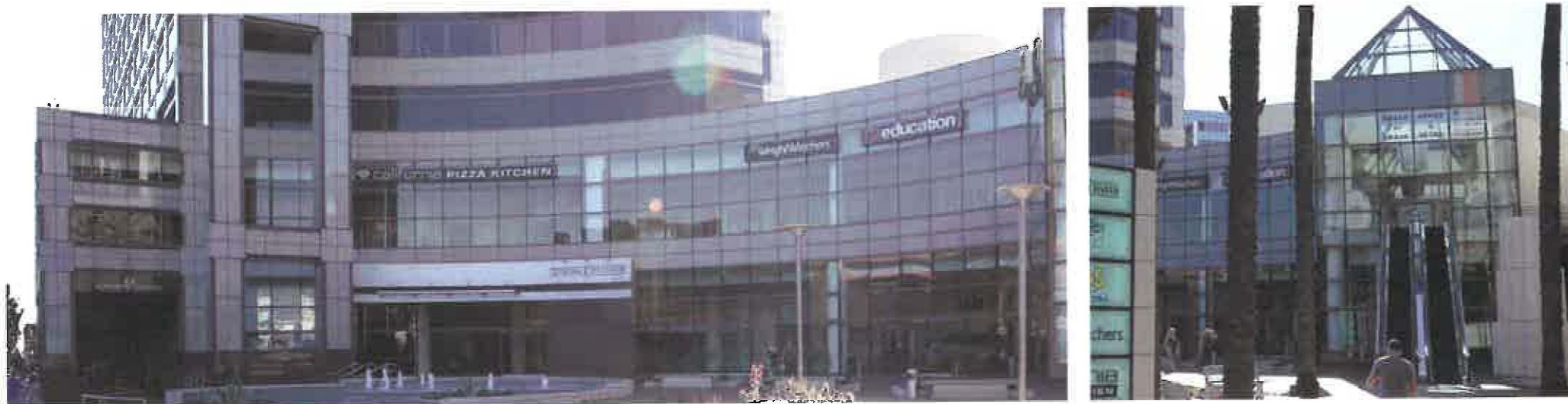
Existing photo of facade/plaza area
