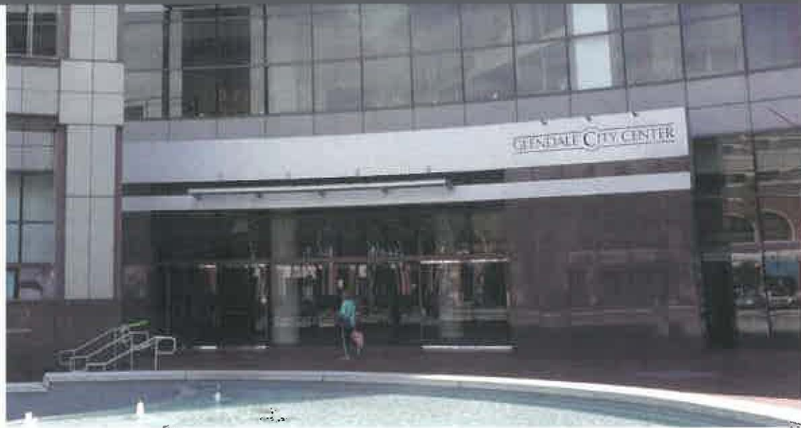
Existing entrance portico with building ID sign
