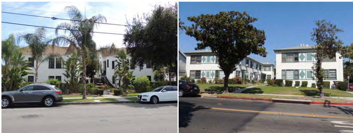
Courtyard apartments representing a variety of architectural styles in the 1930s and 1940s. L: 1118 Lexington, c. 1930. R: 142-146 Adams, 1940. Photographs 2014; Historic Resources Group.
