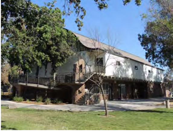
Maple Park Community Building (1966-1967, Arthur Wolfe) with its expressive roof. Photograph 2014; Historic Resources Group.
