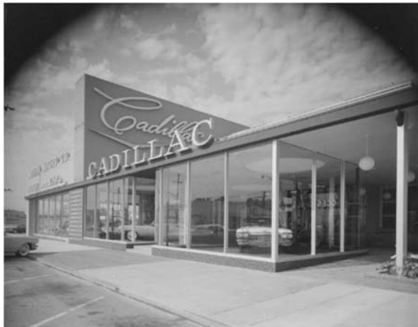
The ultramodern Modern Motors circa 1960 at 1225 S. Brand Boulevard (Heinsbergen Decorating Company) as featured in Architectural Digest in 1960. Photograph: Maynard L. Parker. Source: The Huntington Library Photo Archives.
