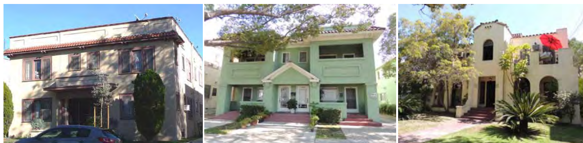
1920s apartment houses in South Glendale, L to R: 618 S. Louise, 106-108 Lomita Avenue, 110 California Avenue. Photographs 2014; Historic Resources Group.
