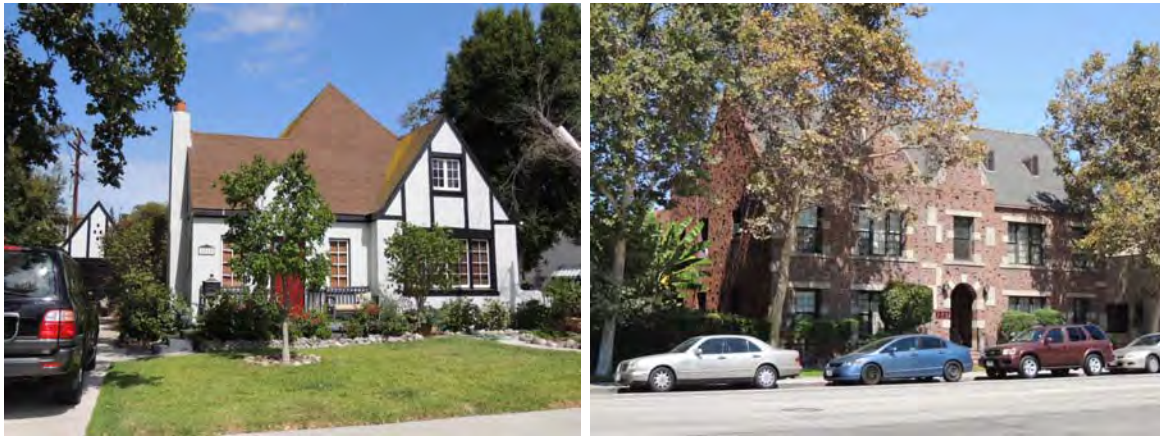
L: 1212 Cottage Grove Dr. (Contributor to Cottage Grove Historic District); R: 1227-1229 S. Central Ave. Source: Historic Resources Group, July 2014.
