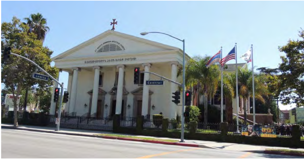
500 S. Central Ave. Source: Historic Resources Group, July 2014.
