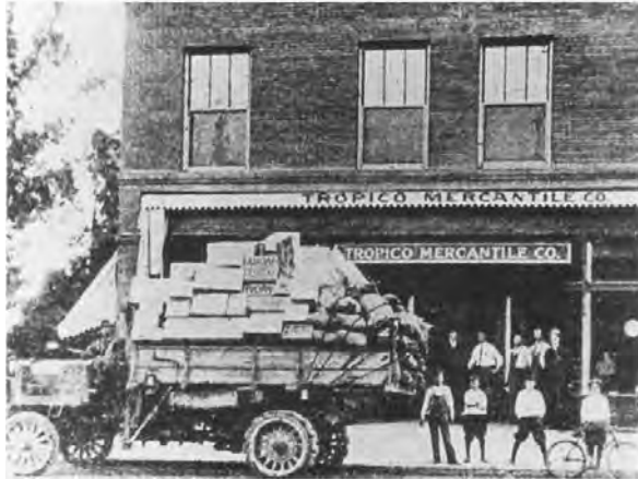
Tropico Mercantile Company (1905) at San Fernando Road and Central Avenue, Tropic. Source: Special Collections Room, Glendale Public Library.
