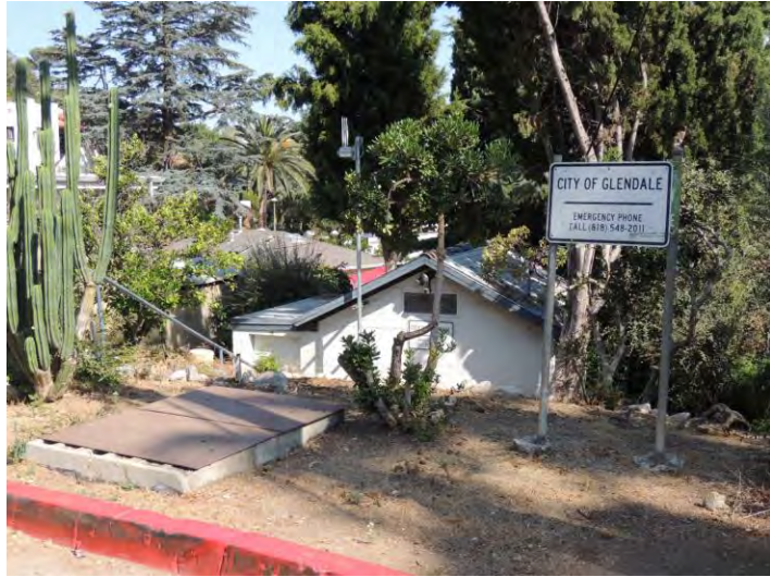
Dartmouth_Dr_1422 (Glendale Heights Water Pumping Station)
