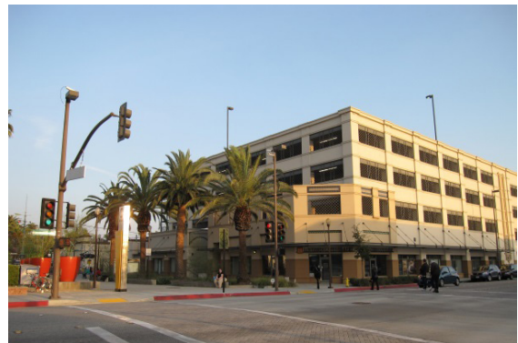
Metro Gold Line Fillmore Station
