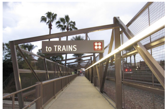
Directional signage at Fullerton Transportation Center
