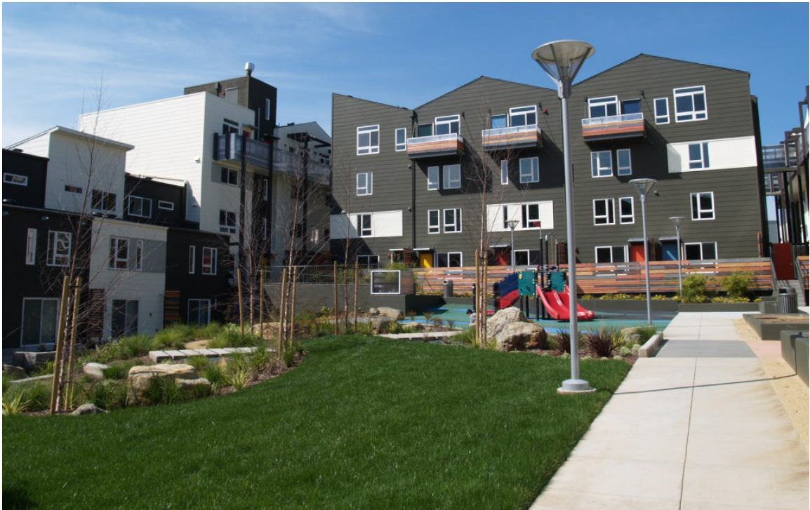
Multi-Family Housing by David Baker Architects, San Francisco
