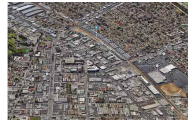
Existing Condition: Birdseye view looking south towards Tropic TOD.
