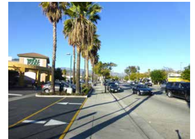
Existing Conditions: View along Glendale Avenue near California Avenue looking north.
