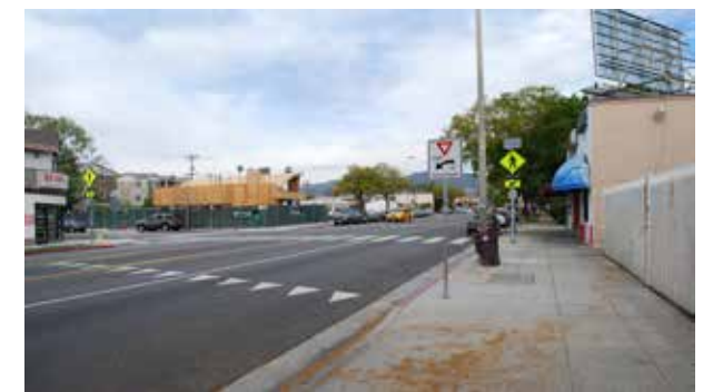
Existing Condition: View along Glendale Avenue near Acacia Avenue looking north
