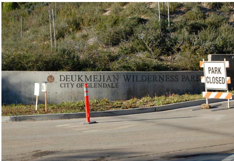
This well-executed sign is part of a retaining wall.
