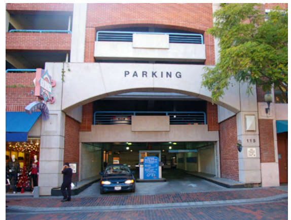
The projecting identity sign, left, is needed, but this elevation needs stronger signage.
