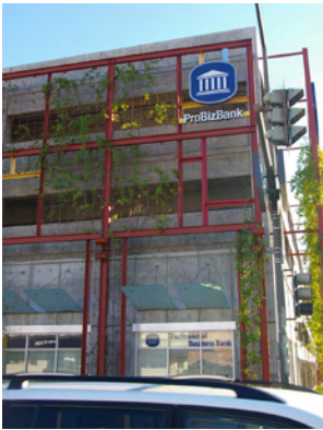
This tenant sign inadvertently identifies the entire parking structure as a private enterprise. The City should have top billing.
