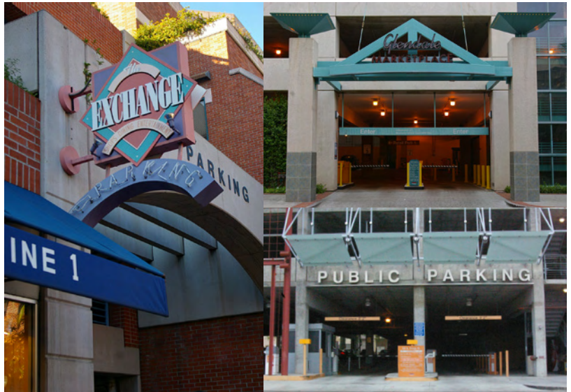
Garage entrances have a variety of sign formats, none of which indicate city ownership or operation.
