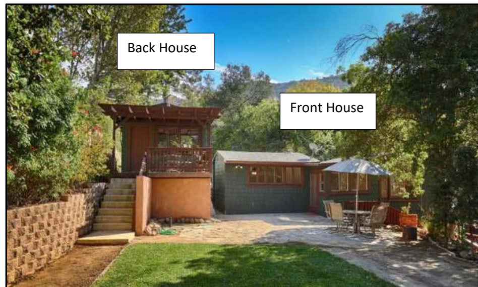
Figure 27. Current Photo of West Facing Elevation
