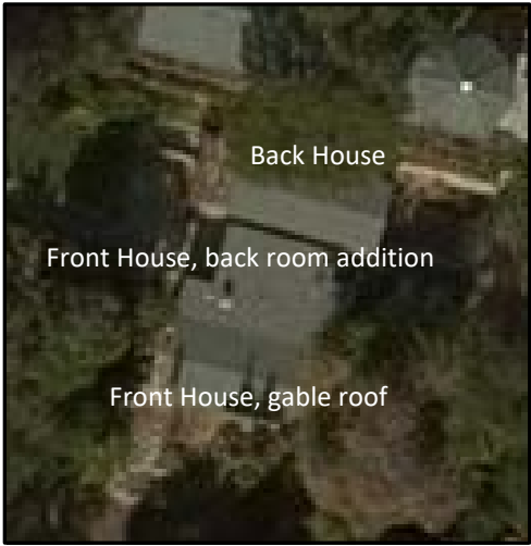
Figure 6. Property Roof View source: Google Maps
