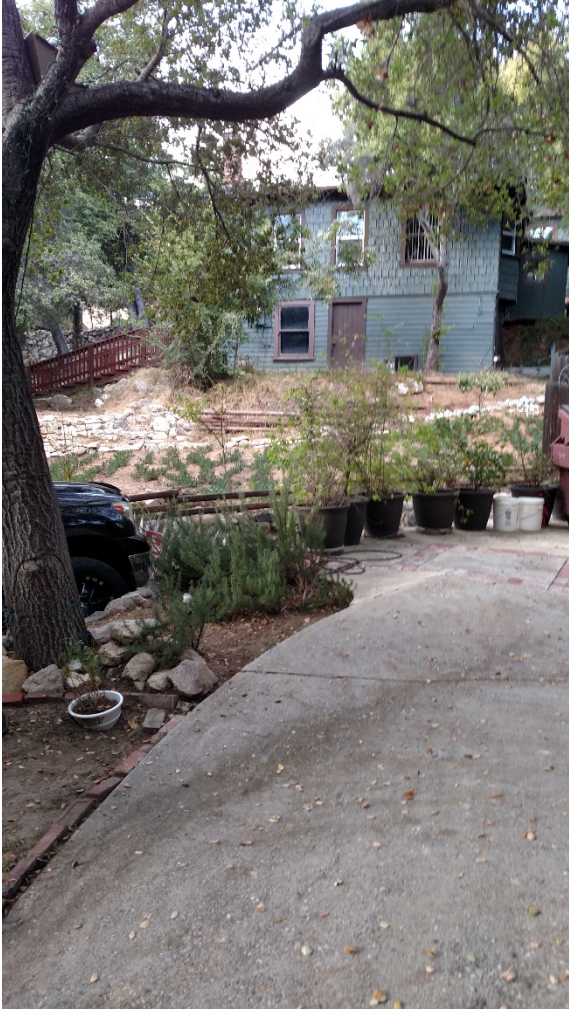
PHOTO 3. A long view of the front home showing the lower basement portion and the upper floor. The lower level is covered in horizontal wood siding and the upper portion is covered in wood shingle siding. An entry door is located on the lower portion.
