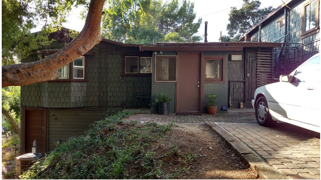
PHOTO 5. Rear view of the front house showing the single-story elevated portion with an enclosed rear porch and a two-story section with a basement area and rear entry built against the hillside slope. A protruding window box, or bay window, is located on the upper floor of this rear elevation. There is no evidence that this portion of the house is a converted garage.
