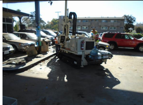
Photograph 8: View of the soil sampling activities at soil boring location SB9.
