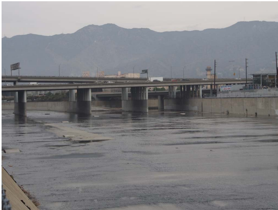
Photo 4: Depicts a thin sheet of flow over the wide, concrete bottom of Segment 2 where the Verdugo Wash enters the Los Angeles River. Photo was taken from the bike path at the southern end of Segment 2 facing north.
