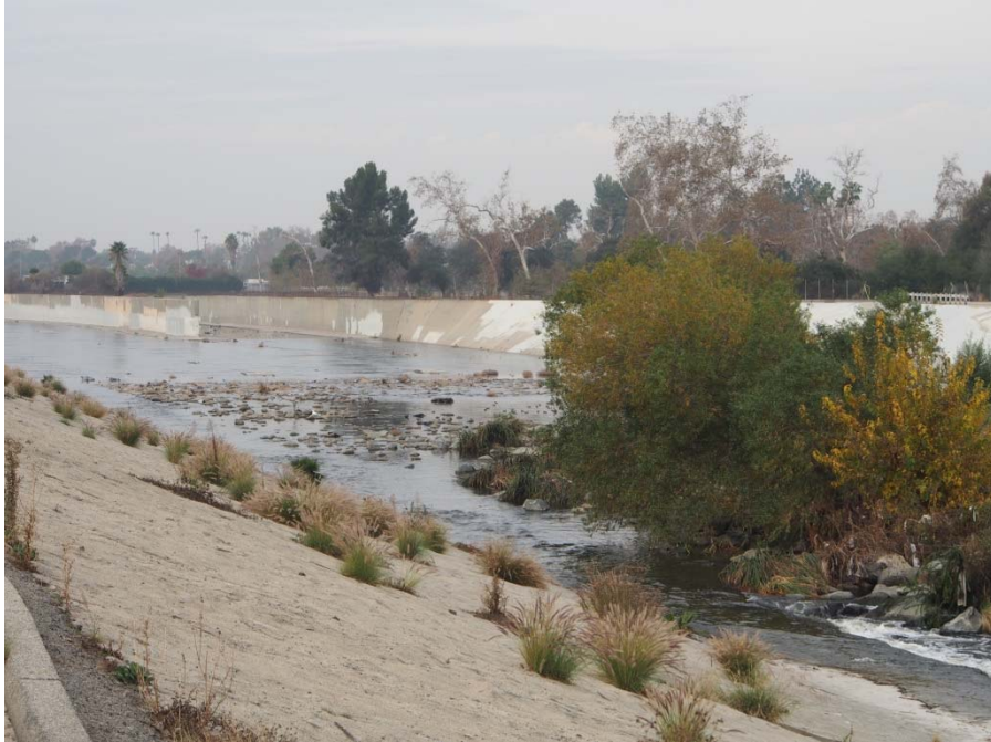
Photo 1: Depicts the outflow from the Burbank Western Channel into the Los Angeles River at the north western edge of the Study Area. Photo was taken from the bike path at the western end of Segment 1 facing northwest.
