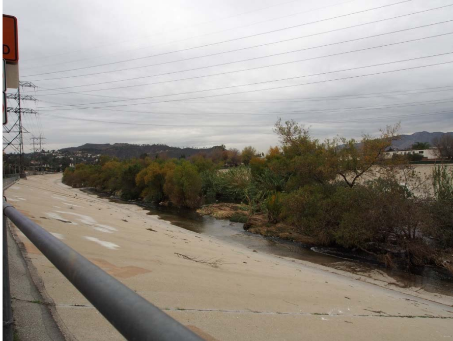
Photo 12: Depicts BWT in the central portion of Segment 4. Photo taken from the bike path facing northeast.
