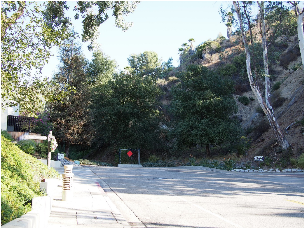
Photo 3: Depicts the road edge where Pump Station #1 is proposed along Chevy Oaks Drive.
