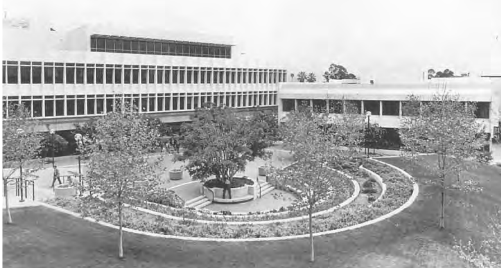
The Landscaped semi-circles of Parcher Plaza at the Glendale Civic Center unify the various civic buildings and provide open spaces for city workers and the public alike. Source: Special Collections Room, Glendale Public Library.
