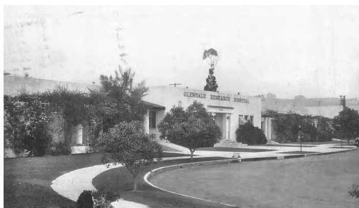
Glendale Research Hospital (1921, Charles W. Kent & Son builders) at N. Adams Street and Doran Drive adjacent to Piedmont Park. The E-shaped plan featured Spanish Colonial Revival pergolas on each side of the main entrance. French doors from all rooms allowed patients to recuperate outdoors. Source: Special Collections Room, Glendale Public Library.
