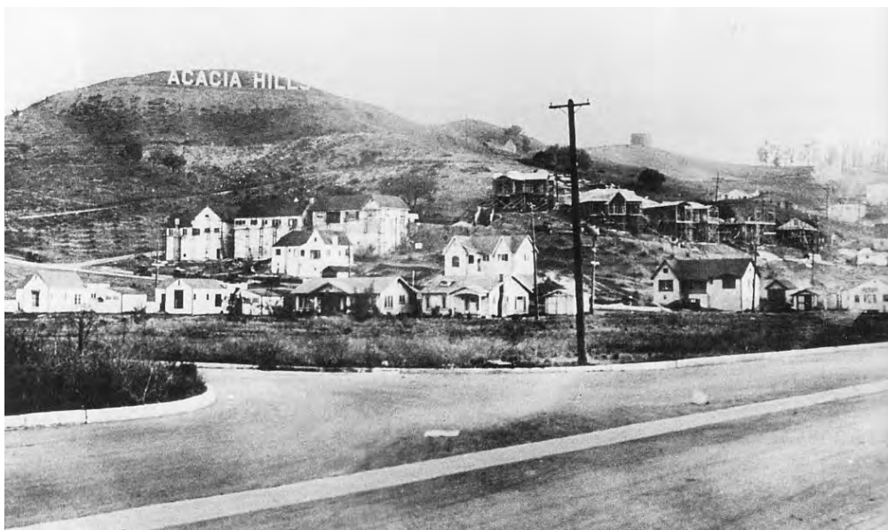
A view of Acacia Hills from Chevy Chase and Garfield Avenue taken around 1925. Note the many undeveloped parcels, as development continued in this area until 1970. Source: Special Collections Room, Glendale Public Library.
