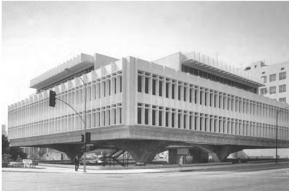
The Glendale Municipal Services Building (1966, Merrill W. Baird and A.C. Martin & Associates) floats fourteen feet above ground level on four pylons. It is Glendale Register #100. Source: Special Collections Room, Glendale Public Library.
