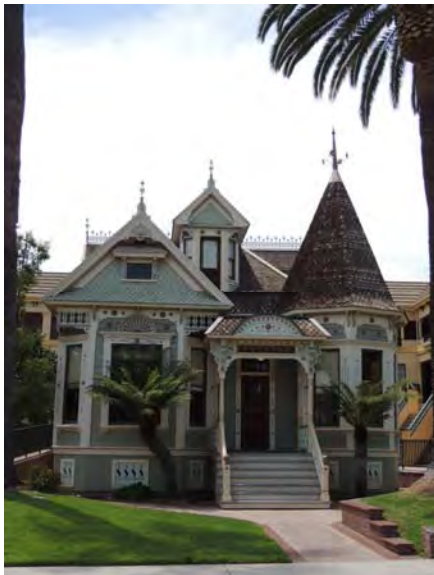
119 N. Cedar St., E. D. Goode House (Glendale Register #8). Source: Historic Resources Group, July 2014.
