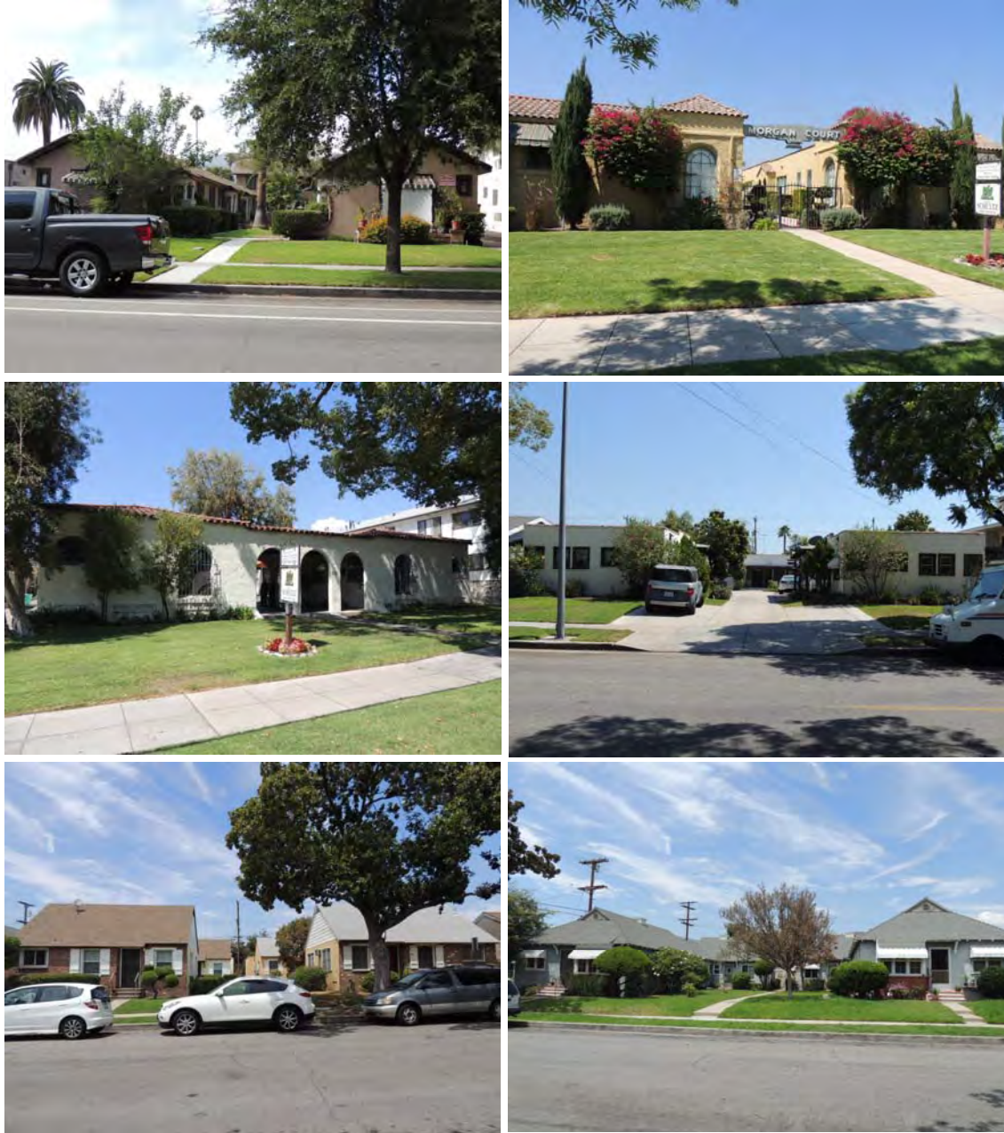
One-story courts in a variety of architectural styles, including a small cluster along California Avenue. TL: 415 Riverdale, 1923. TR: Morgan Court, 1119-1123 California Avenue, c.1925. ML: 1129-1131 California Avenue, 1927. MR: 1136 California Avenue, 1922. BL: 1423 Barrington Way, 1941. BR: 1415 Barrington Way, 1942. Photographs 2014; Historic Resources Group.
