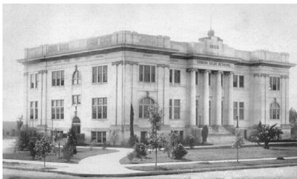
Glendale Union High School (1908, Norman F. Marsh) was located at 210 E. Harvard Street. Clad in buff pressed brick it held a 450-person auditorium. Source: Special Collections Room, Glendale Public Library.
