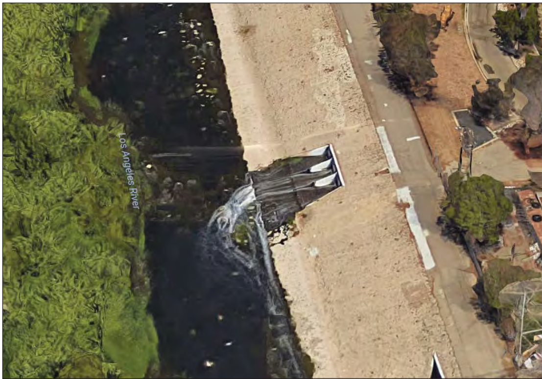
PHOTOGRAPH 1: Los Angeles River at LAGWRP Discharge Point
