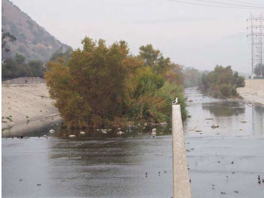
Photo 7: Depicts the BWT at the southern end of Segment 3. Photo was taken from Los Feliz Boulevard facing north.
