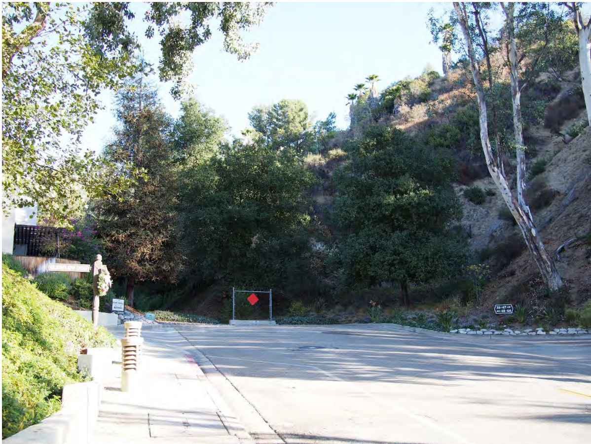
Photo 3: Depicts the road edge where Pump Station #1 is proposed along Chevy Oaks Drive.
