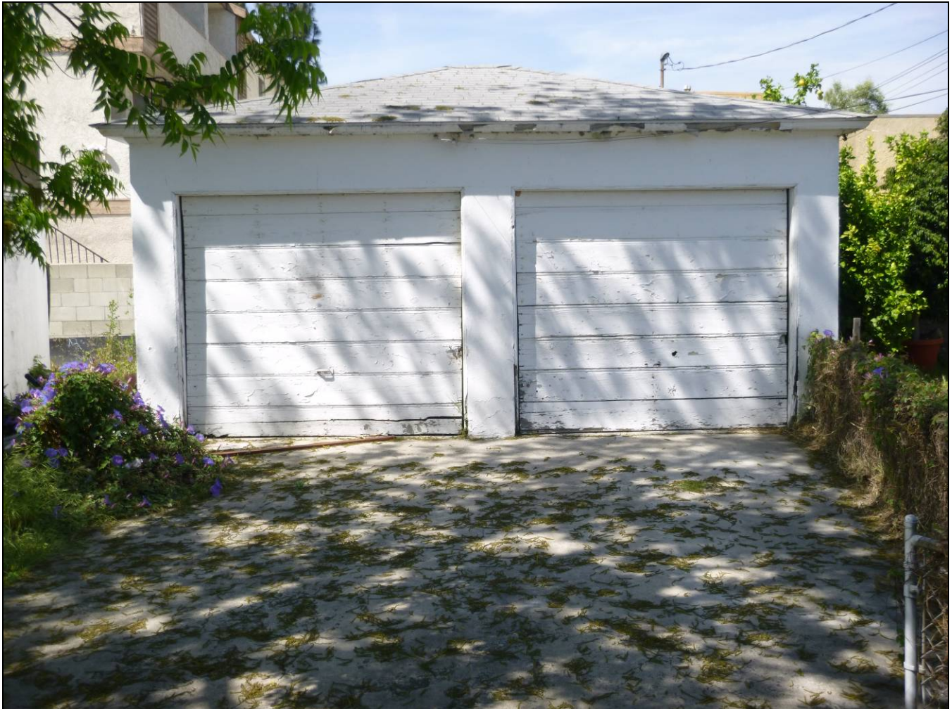
Detached two-car garage to the rear (north) of the residence at 405 Hawthorne Street (view to the north; photograph taken April 21, 2016).
