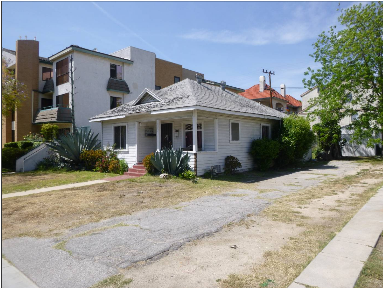
South and east elevations of the Transitional Craftsman style single-family residence at 409 Hawthorne Street (view to the northwest; photograph taken April 21, 2016). The asphalt driveway leads to a small automobile-house at the rear of the parcel.
