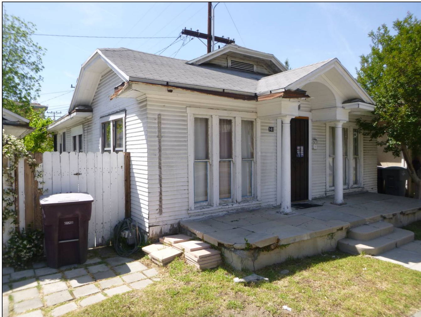
South and east elevations of the Colonial Revival single-family residence at 141 S. Columbus Avenue (view to the northwest; photograph taken April 21, 2016).
