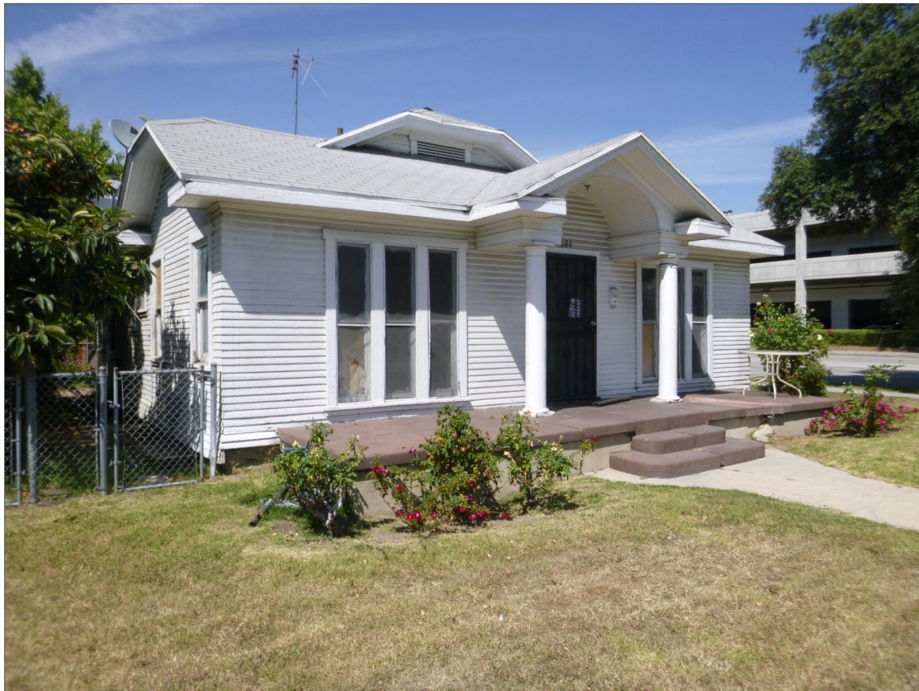
South and west elevations of the “Clipped-Gable Colonial” single-family residence at 401 Hawthorne Street (view to the northeast; photograph taken April 21, 2016).
