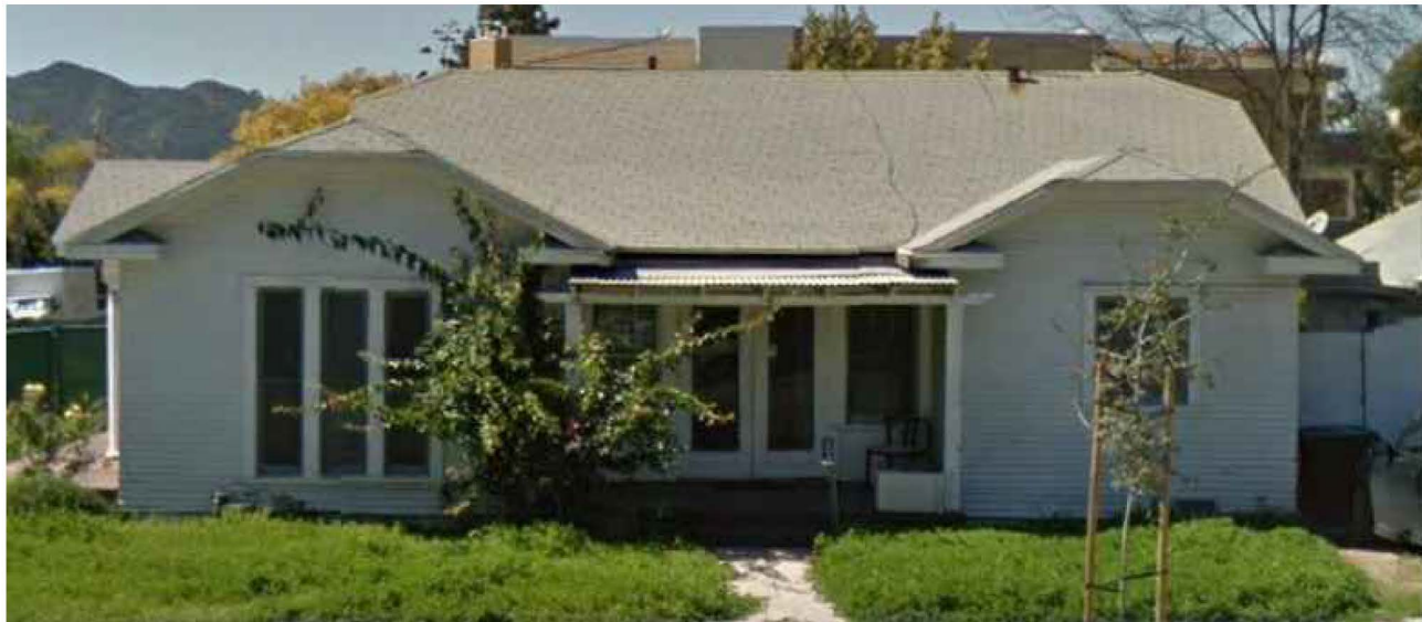
HOUSE 401 EAST ELEVATION—EXISTING
