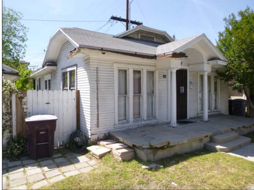
Figure 6 South and east elevations of 141 Columbus Avenue (view to the west; photograph taken April 21, 2016).
