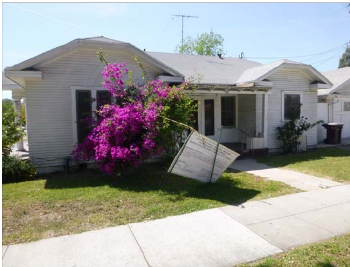
Figure 8 East elevation of 401 Hawthorne Street (view to the north; photograph taken April 21, 2016).
