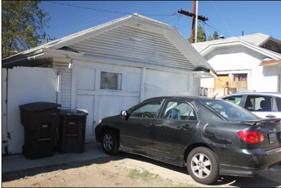
Figure 9 Exterior shared garage (view to the west; photograph taken November 11, 2016).
