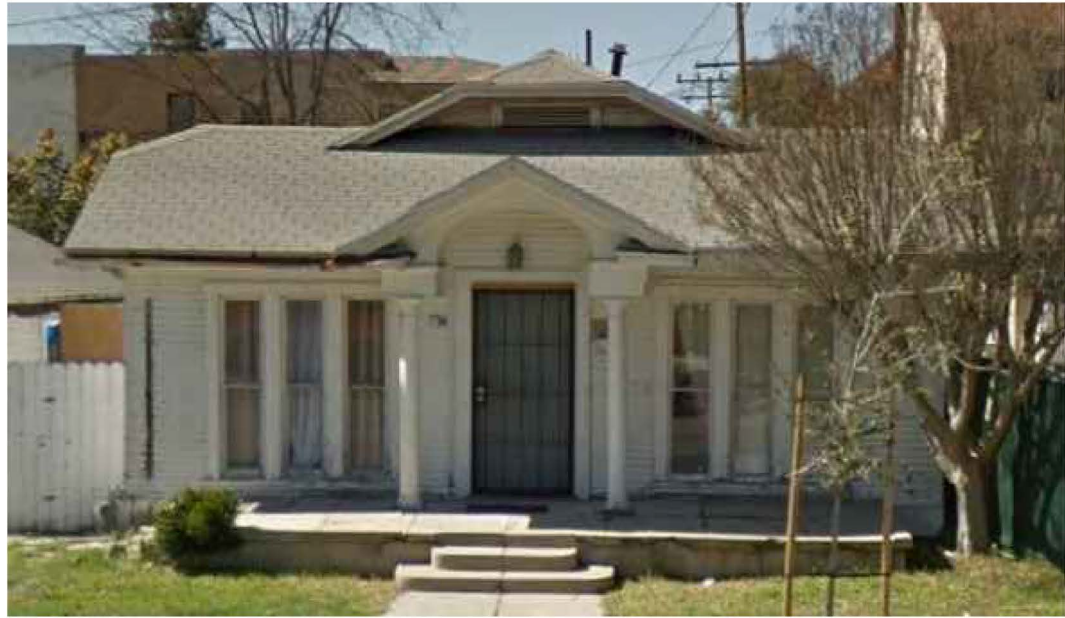
HOUSE 141 EAST ELEVATION—EXISTING
