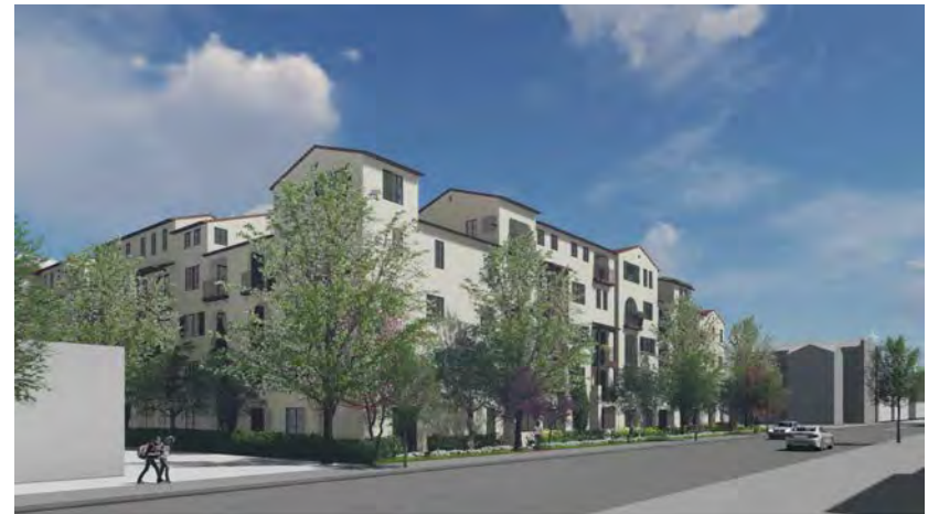
VIEW LOOKING SOUTH ALONG KENWOOD ST
