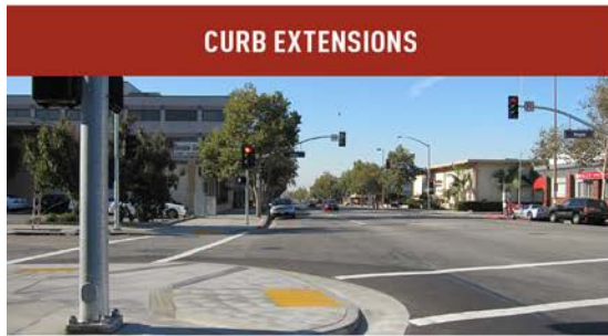
Curb extension in downtown Glendale Photo from the City of Glendale
