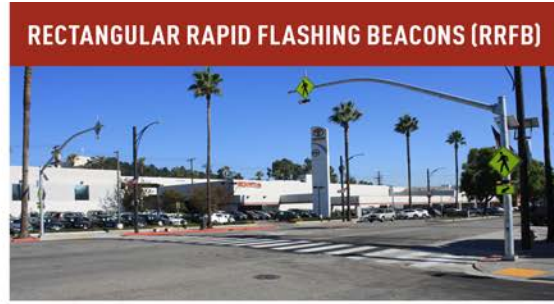
RRFB in Glendale Photo from the City of Glendale
