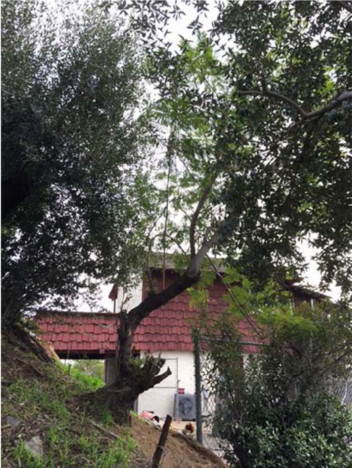
Figure 9: Looking southeast at Tree 8. This tree will not likely be impacted by construction. It was severely pruned in the past.
