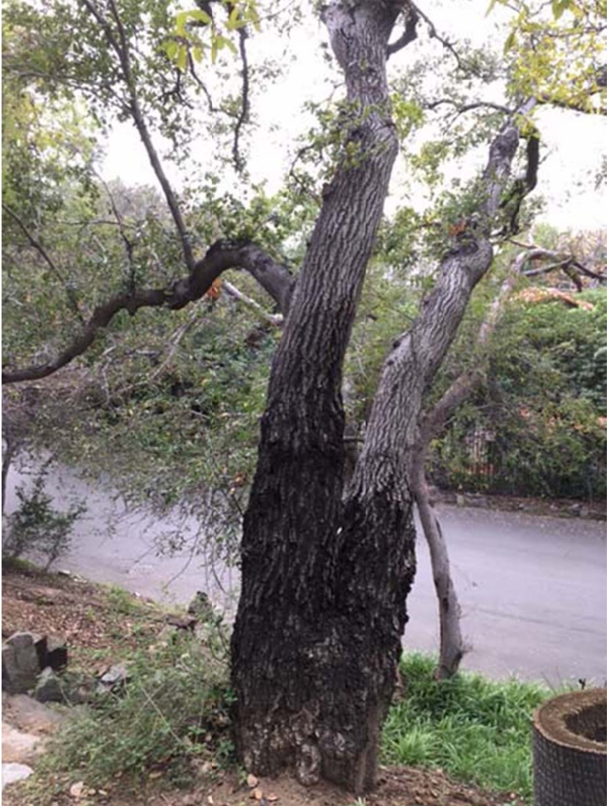
Figure 15: Looking west at Tree OP14. This tree is intended for preservation through construction. It has signs of bark beetle infestation in the lower trunk.
