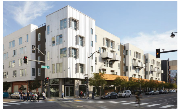
ABOVE: Major and minor building facade modulations can create depth and scale.
