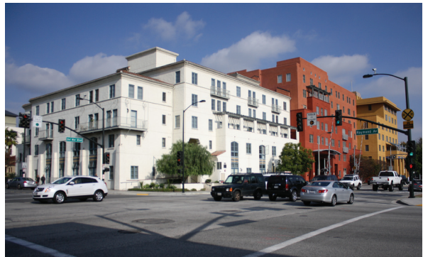
ABOVE: Height averaging allowed for variations in massing to locate a taller building and corner tower feature addressing a wide, high-traffic street, and stepped down massing facing lower height buildings and a public park.
