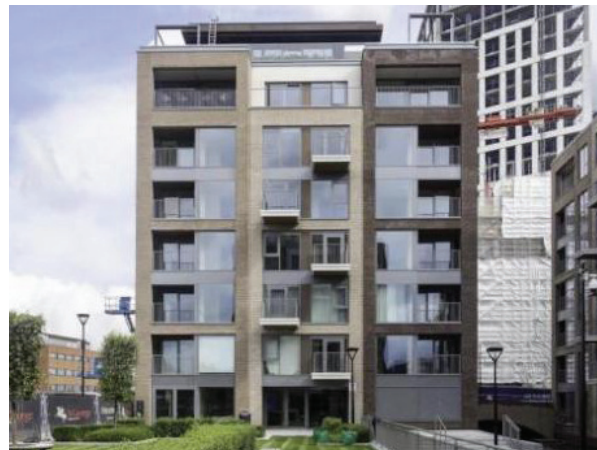
ABOVE: A mix of recessed and partially recessed balconies can create visual interest and articulation in facades.
