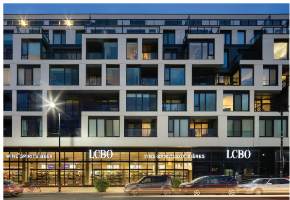
ABOVE: Recessed balconies can be incorporated into a facade design to create a unique pattern or form.
