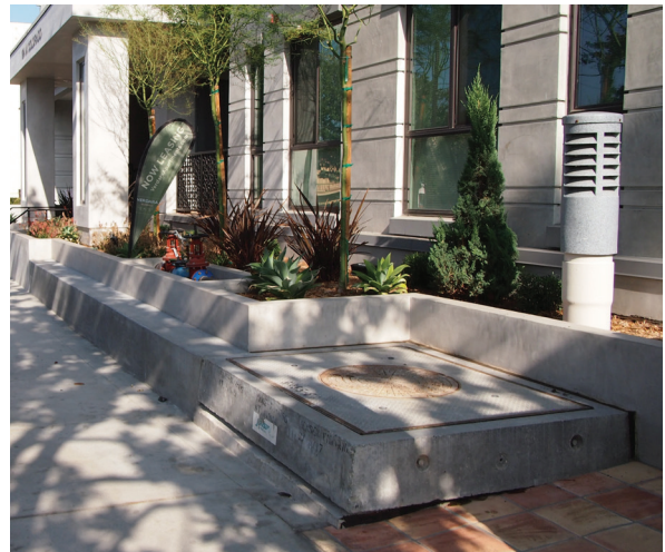
ABOVE: Utilities shall not interrupt the design of planters or other building elements, unlike the photo above. They shall be gracefully integrated into the overall design and shall be accounted for early in the design process to avoid negative visual impacts.
