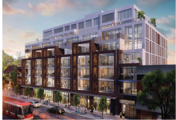
ABOVE: Upper level building stepbacks can reduce the scale of a building and improve its relationship to the pedestrian realm.
