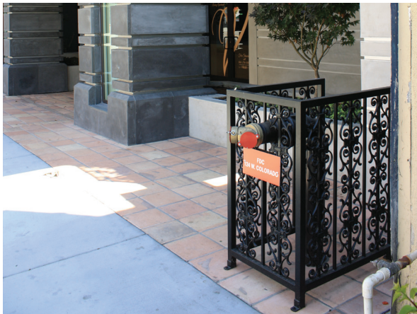
ABOVE: When utilities must project from the building facade at the pedestrian level, they shall be enclosed with an architecturally compatible surround to prevent tripping hazards and to improve the aesthetic impact.
