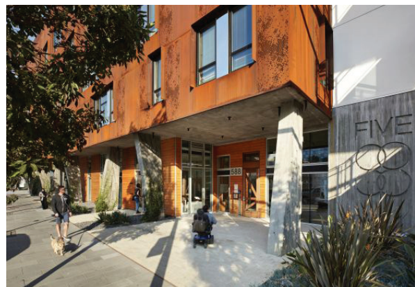
ABOVE: Recessed entries can create modest open spaces and differentiation in the street frontage.
