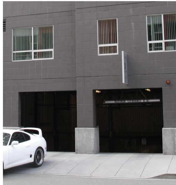
ABOVE: Narrow garage entry widths encourage slower movement of automobiles reducing potential conflicts with other modes of transportation.
