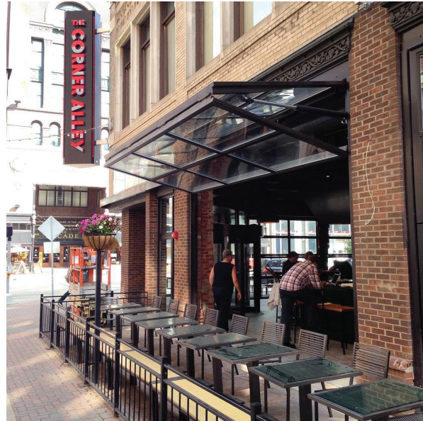
ABOVE: Doors and windows that fold and swing can create a unique aesthetic in an urban environment. They engage the public realm with commercial and retail activities by creating permeability in the facade and opportunities for engagement between patrons and passersby.
