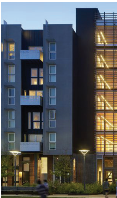
ABOVE: Partially recessed balconies, when combined with major facade modulations can create breaks in large building masses to reduce the overall building scale.
