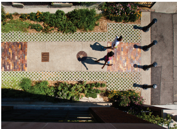
ABOVE: A paseo (plan view) with a creatively designed paving pattern that transitions from inground planted edges - to open-celled concrete pavers - to alternating bands of running course brick pavers and concrete.
