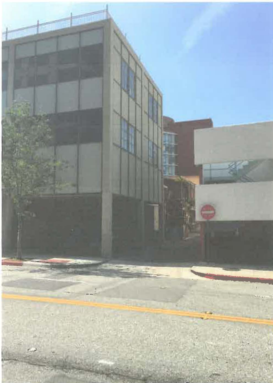
WEST ELEVATION SUBJECT PROPERTY: 429-431 NORTH BRAND BOULEVARD
