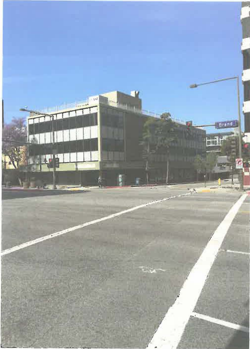
NORTH ELEVATION SUBJECT PROPERTY: 429-431 NORTH BRAND BOULEVARD
