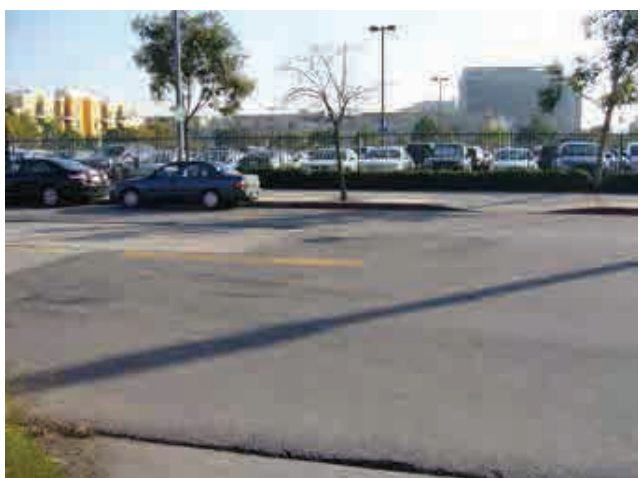
3.8 Fenced parking is a barrier for community access
