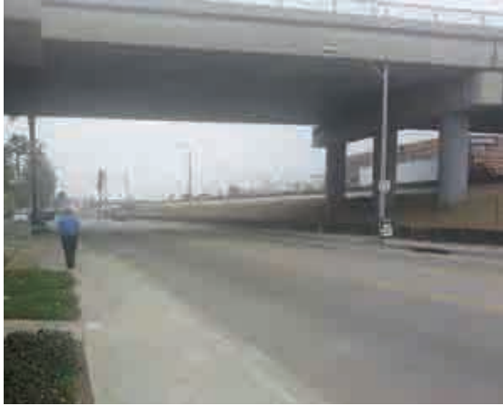
1.1/1.6 No pedestrian lighting adjacent to Metrolink/cut through traffic at unsafe speeds.
