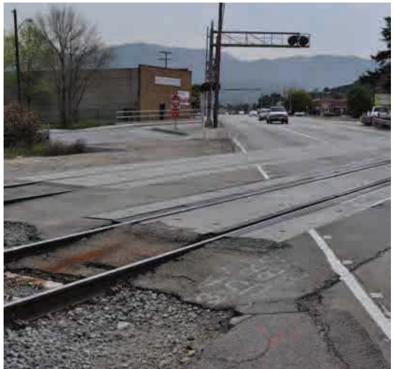
3.2 Non-accessible pedestrian path across tracks
