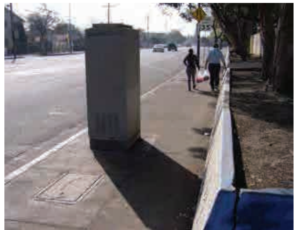
3.1 Utility obstructions in sidewalk right-of-way
