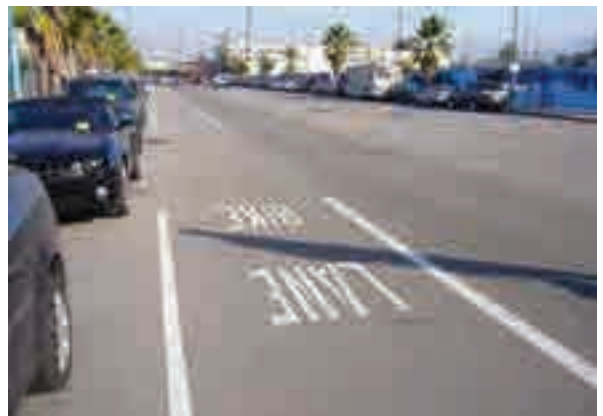
Lack of crossings along superblocks and bike facility without special markings or enhancements
