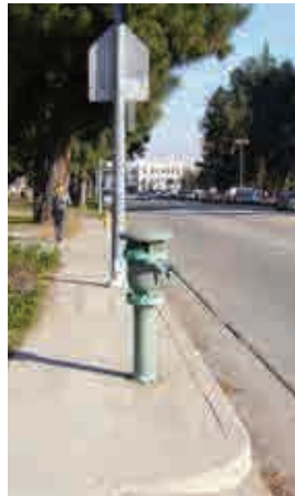
3.1 Utilities in sidewalks
