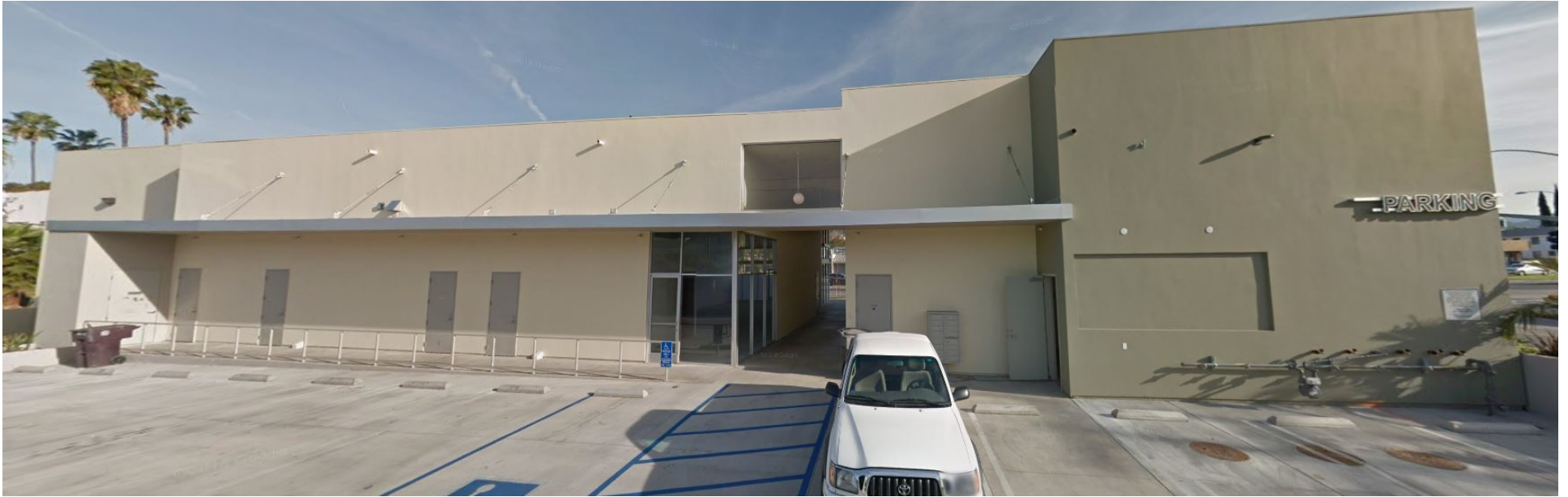
SOUTH FAÇADE - ALLEY
