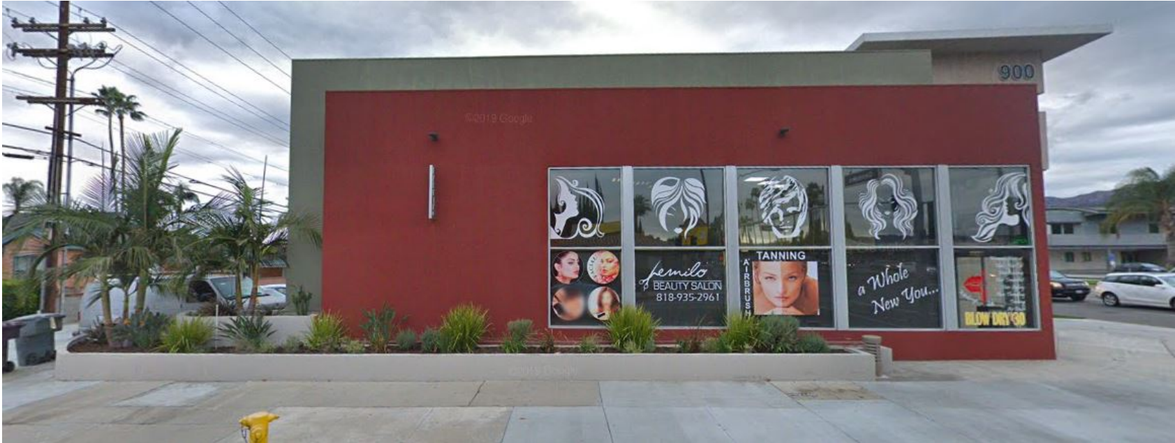
EAST FAÇADE – HIGHLAND AVE.
