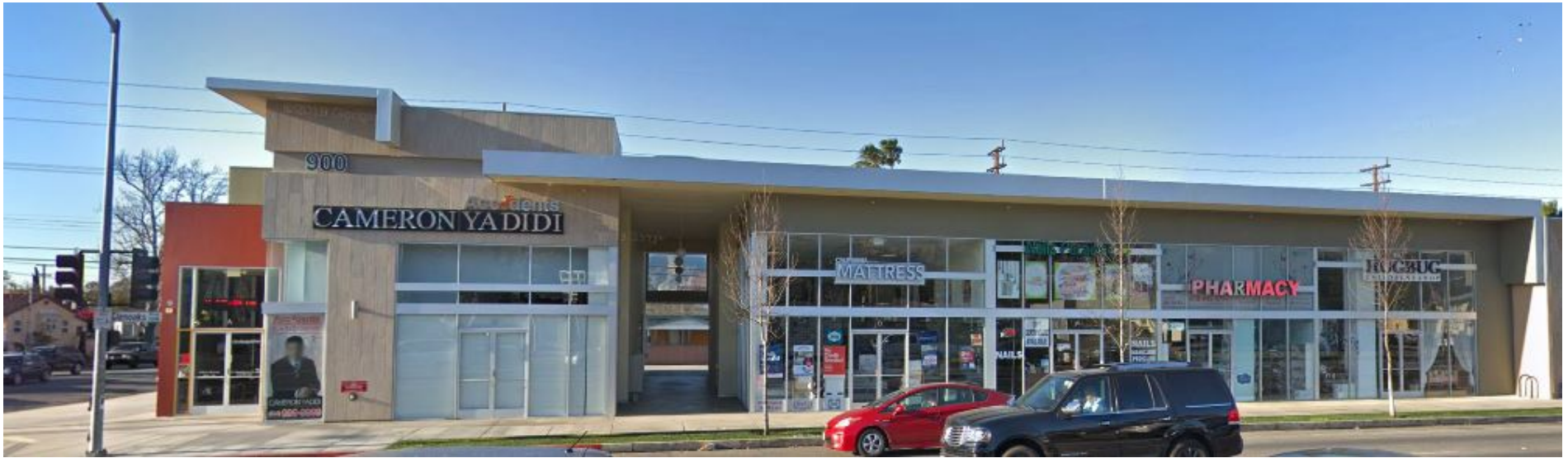
NORTH FAÇADE – MAIN ENTRANCE GLENOAKS BLVD.
