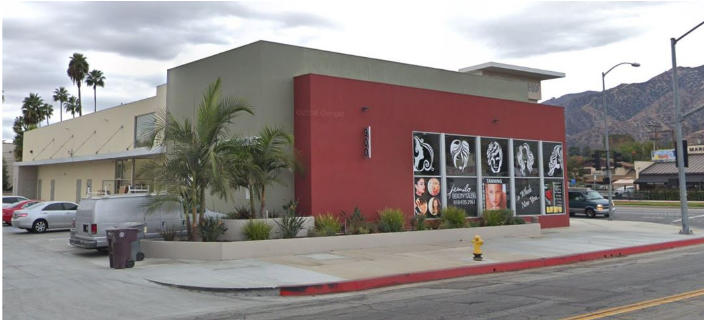
SOUTH EAST CORNER
