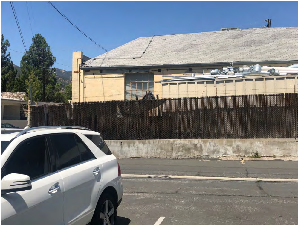
3450 VERDUGO RD. ( WEST PROPERT LINE, FACING ALLEY.)
