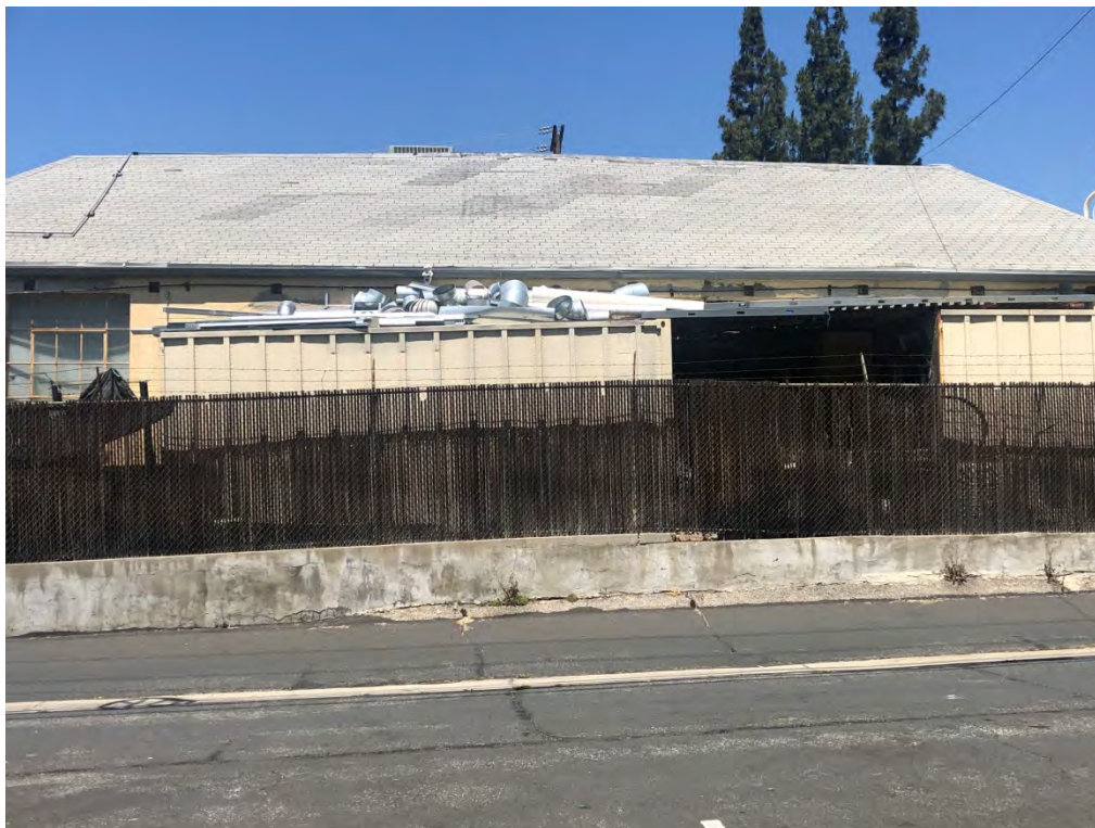
3450 VERDUGO RD. (WEST PROPERT LINE, FACING ALLEY.)
