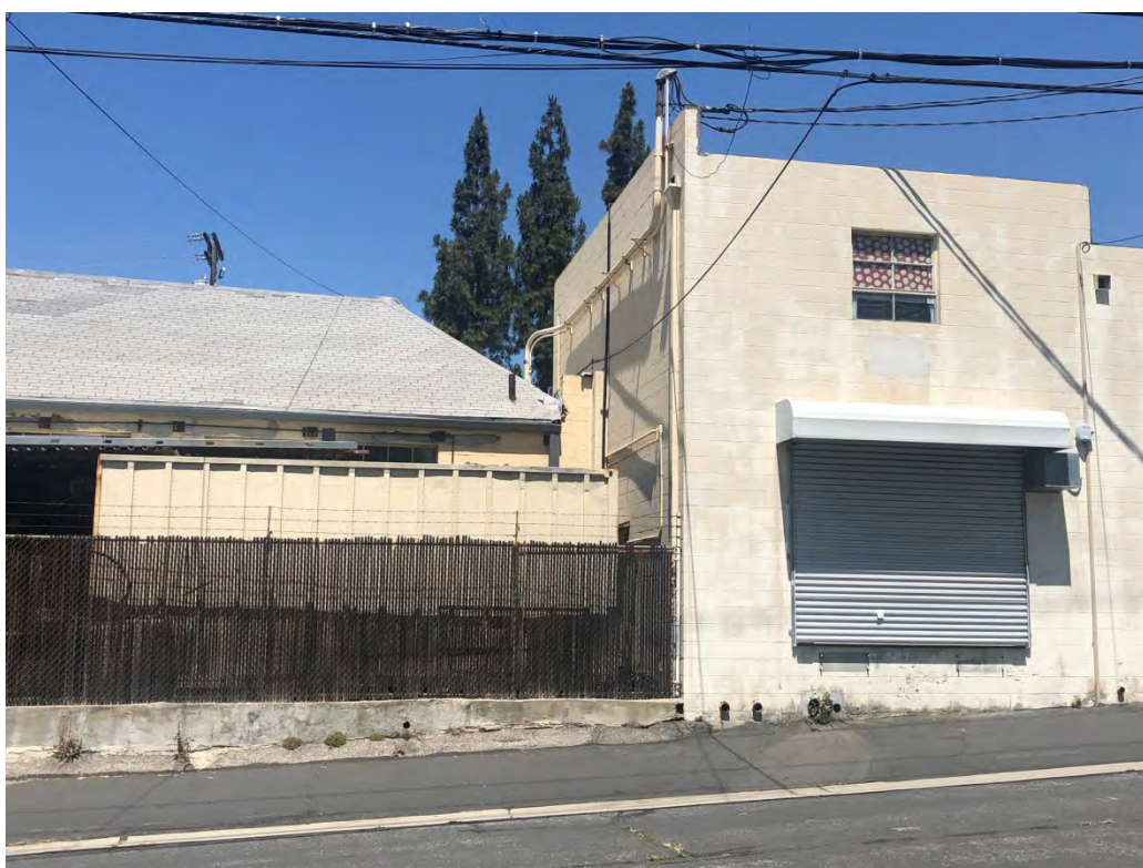
3450 VERDUGO RD. (WEST PROPERT LINE, FACING ALLEY.)
