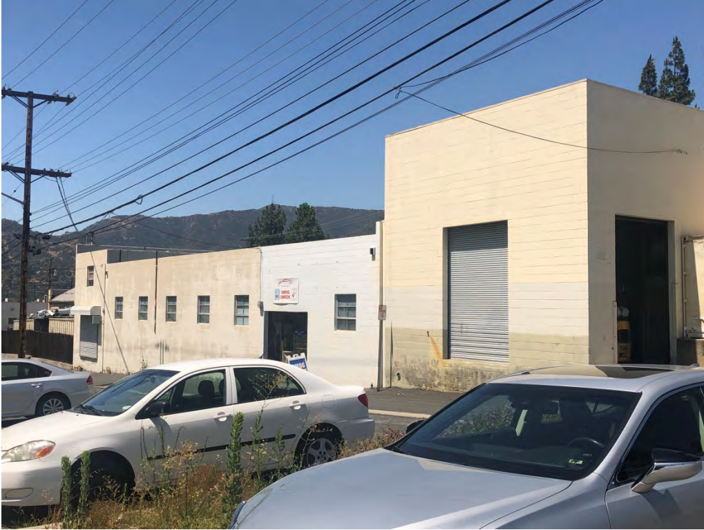
3450 VERDUGO RD. (WEST PROPERT LINE, FACING ALLEY.)
