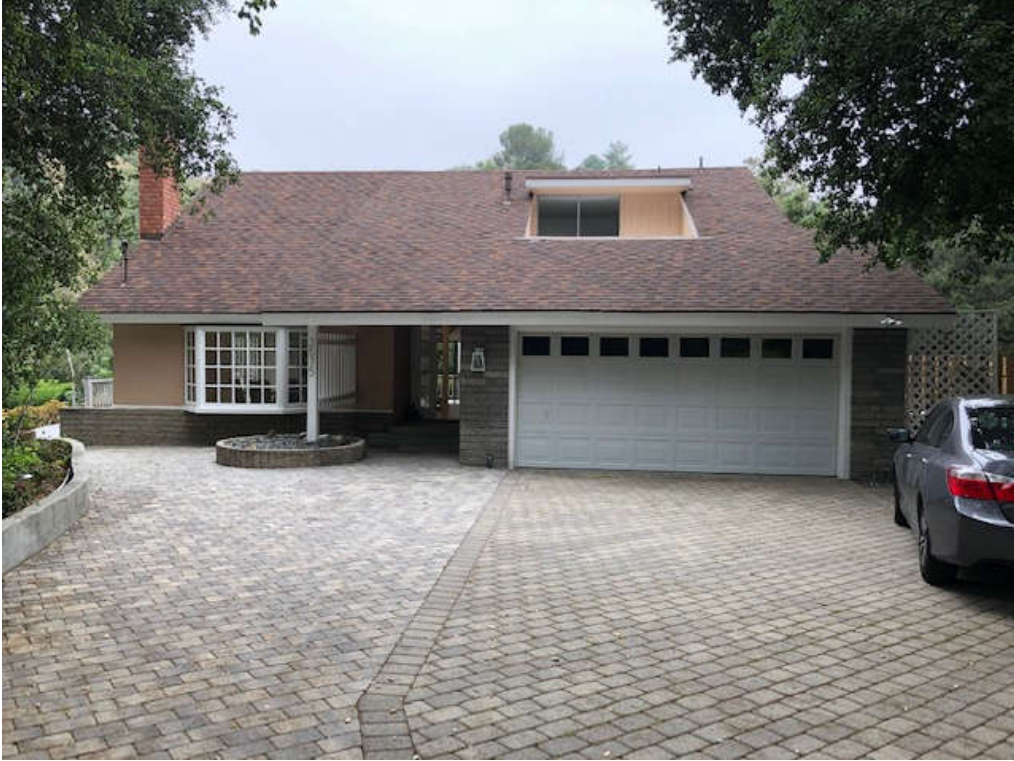
View from the South (entrance)
