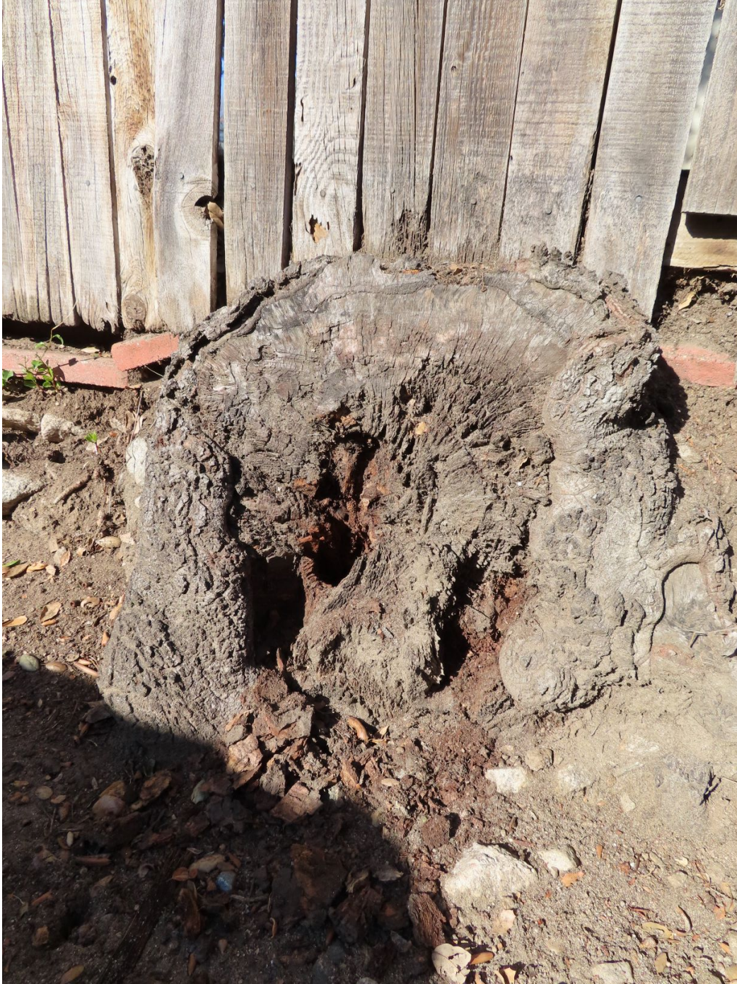
View of the cavity opening at the removed trunk base.
