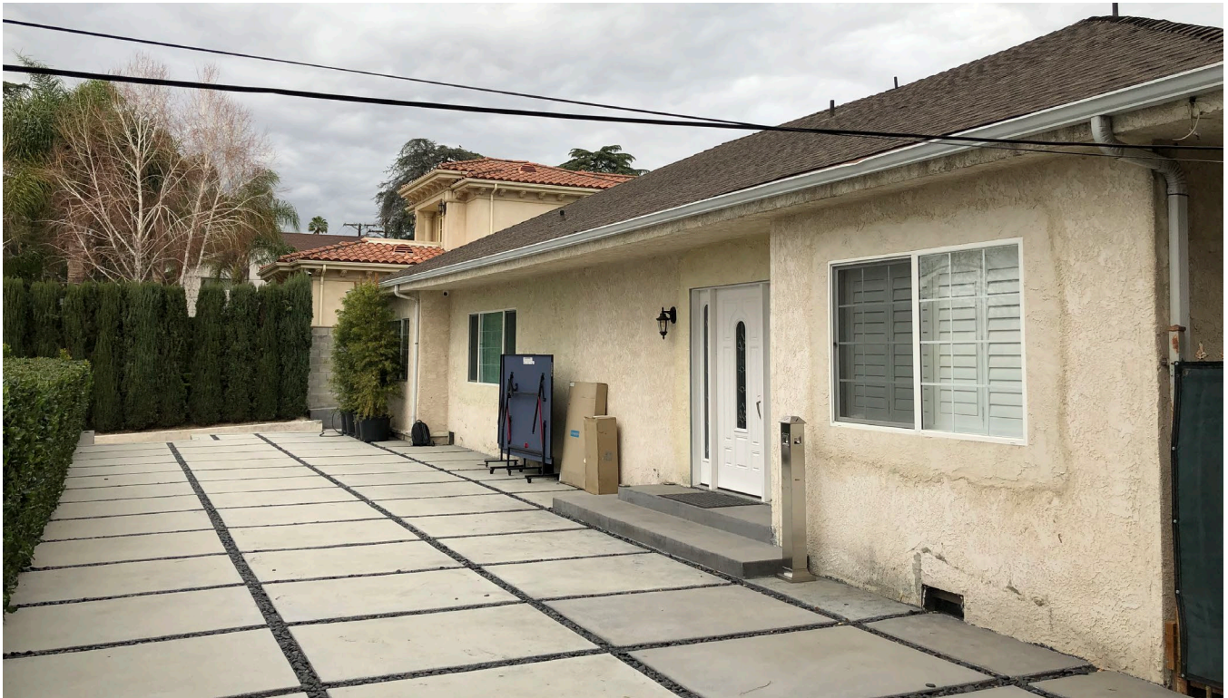
2) MAIN FAÇADE NORTHWEST
