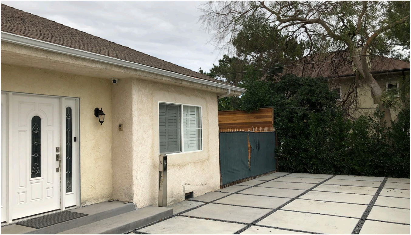
1) MAIN FAÇADE SOUTHWEST
