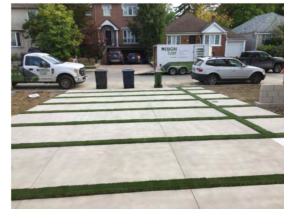
CONCRETE DRIVEWAY WITH ARTIFICIAL GRASS STRIPS
