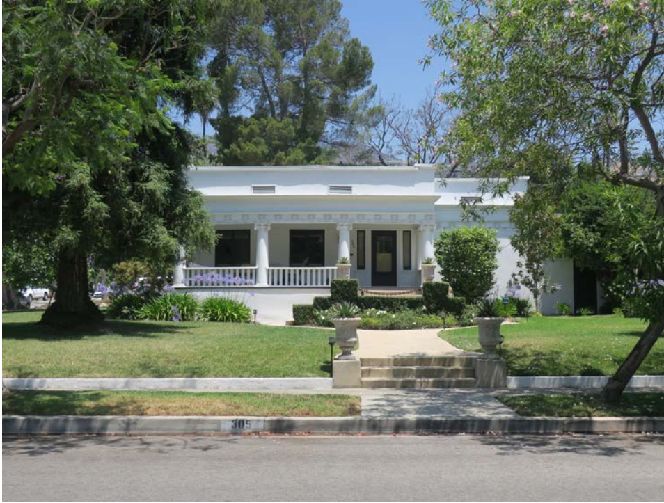
Figure 8. Newton House, 305 E. Randolph Street, built in 1906 and listed in the Glendale Register of Historic Resources. Photo by ARG
