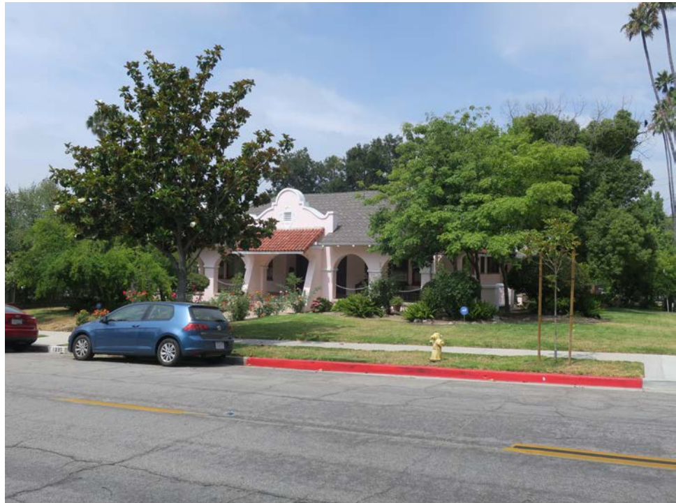
Figure 7. Casa Verdugo, 1235 N. Louise Street, built in 1907 and listed in the Glendale Register of Historic Resources. Photo by ARG
