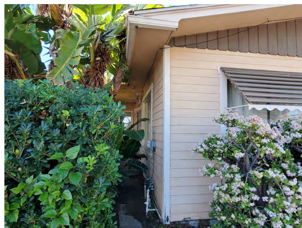
VIEW FROM WEST MILFORD ST
