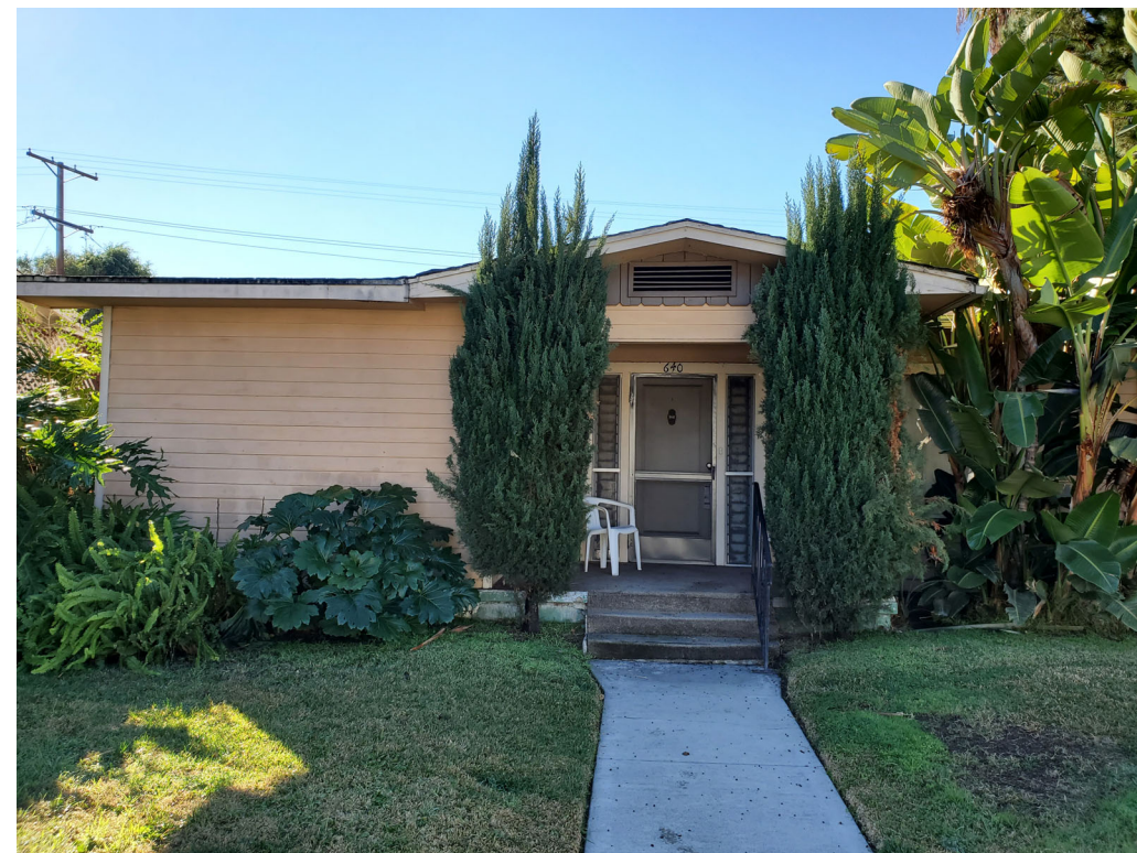
VIEW FROM WEST MILFORD ST
