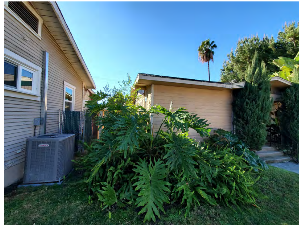
VIEW FROM WEST MILFORD ST
