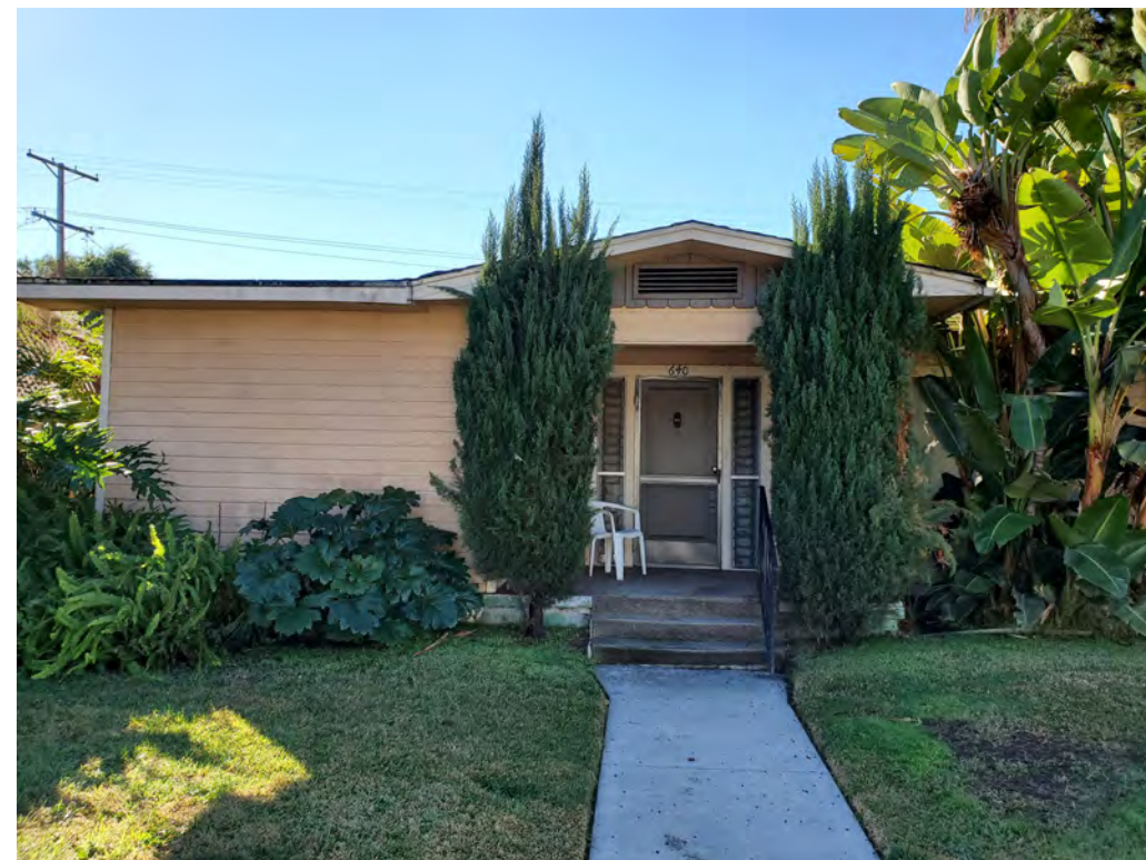
VIEW FROM WEST MILFORD ST
