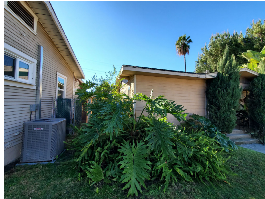
VIEW FROM WEST MILFORD ST
